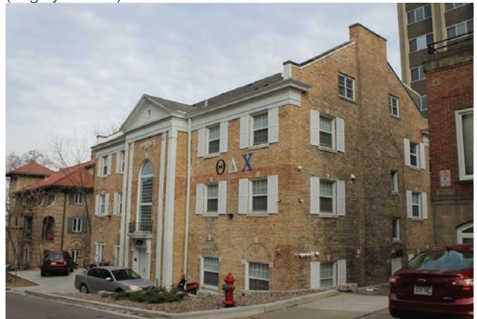
IMAGE 29: The original Georgian Revival Theta Chi Fraternity House built at 144 Langdon Street in 1924-25.
