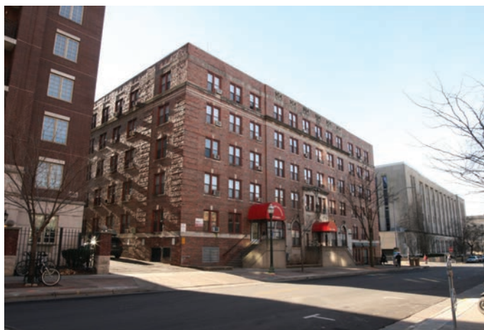
IMAGE 20: Large-scale apartment building at 633-635 Langdon Street.
