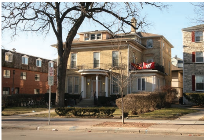
IMAGE 27: The Italianate style Sloan-Ogilvie House at 234 Langdon Street was built in 1875-76 and remodeled as a fraternity in 1928.
