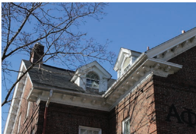
IMAGE 43: End gable moldings and dormers are prevalent throughout the district as seen here at 28 Langdon Street.
