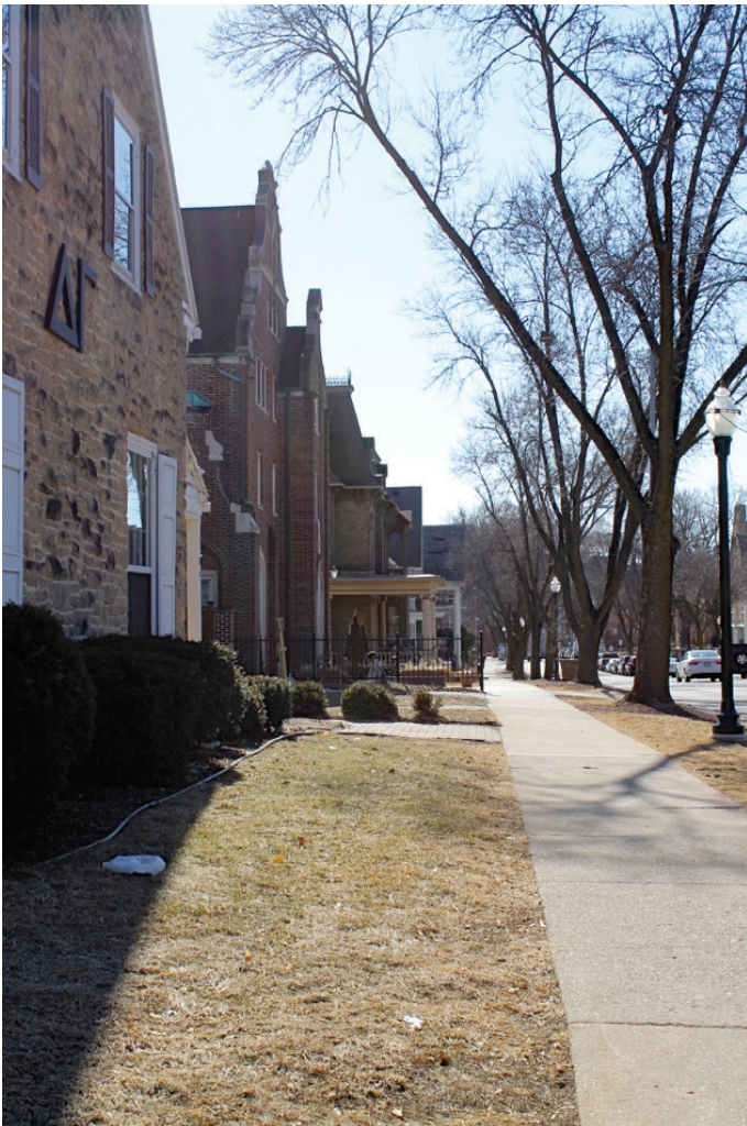
IMAGE 17: Uniform street setbacks and terraces at North Carol Street north of Langdon Street.
