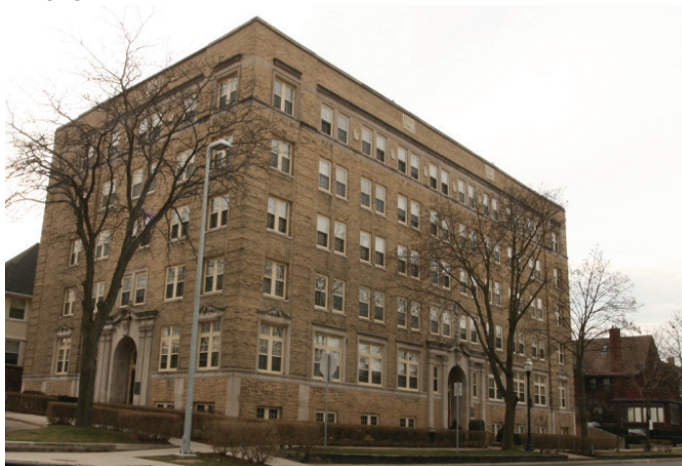
IMAGE 33: The Neo-Classical Revival Kennedy Manor Apartments at 1 Langdon Street was built in 1929.
