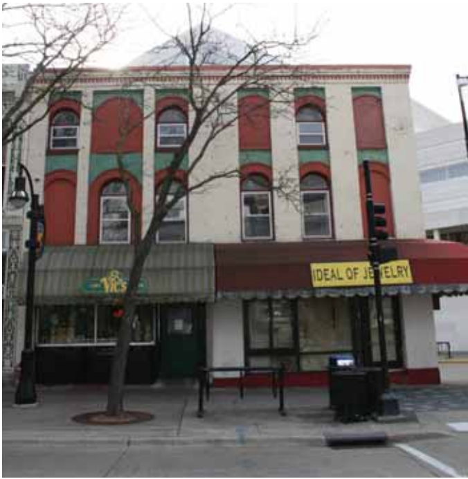
View of Front Facade
