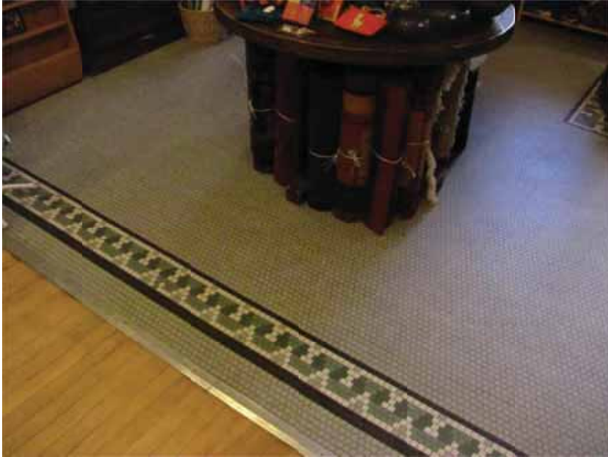
Figure 15. Hardwood and mosaic ceramic tile flooring in the first floor retail space.
