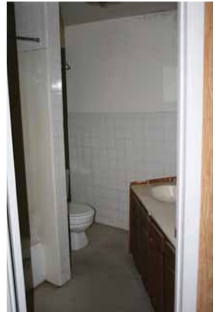
Third Floor: Bathroom
