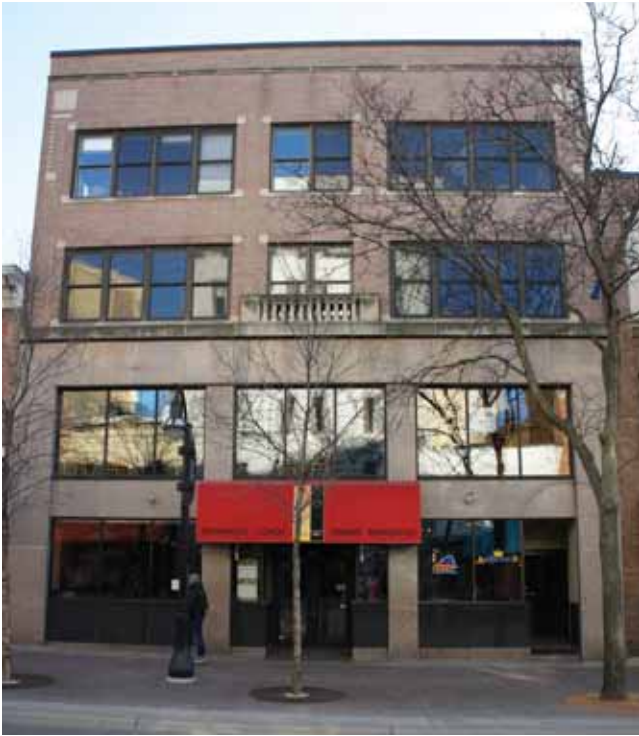
View of Front Facade
