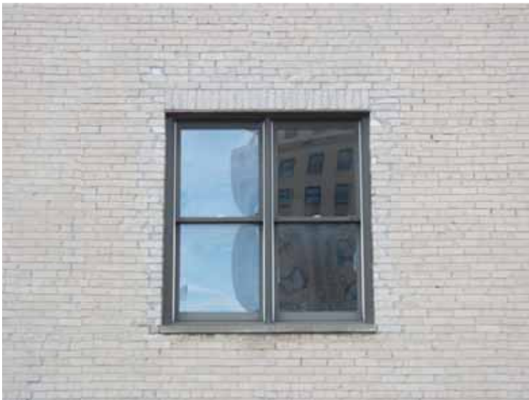
Figure 9. Typical aluminum-clad wood windows.
