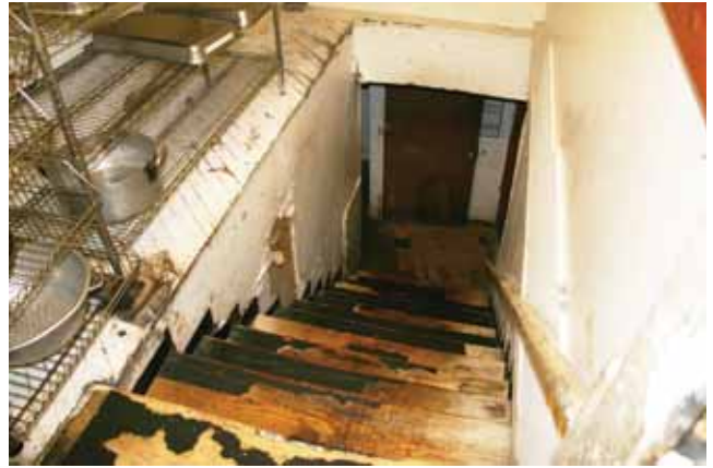
First Floor: View of access to basement
