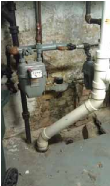
Building service entrances
