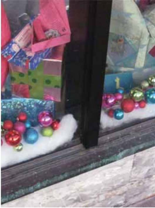
Figure 6. An aluminum mullion has been added at the center of the storefront at the first floor of the State Street facade.
