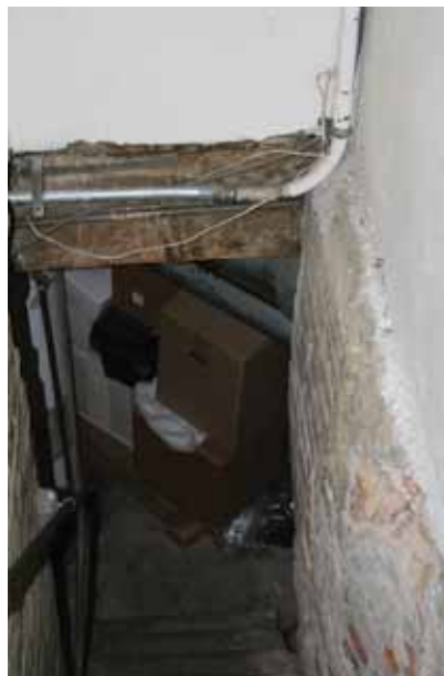
Basement Access Stair
