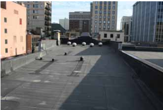
Roof view toward Mifflin Street
