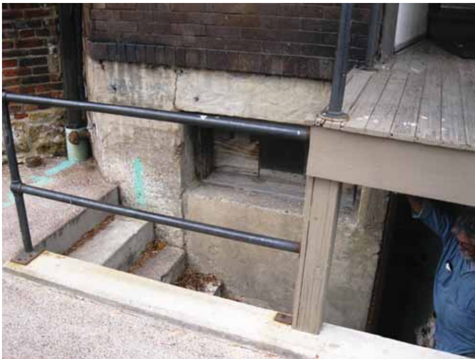
Photo 4 – Stair to basement from Fairchild Street
