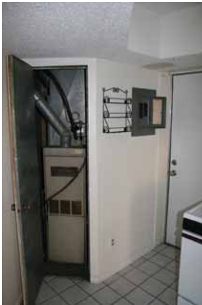
Second Floor: Mechanical and door to fire escape
