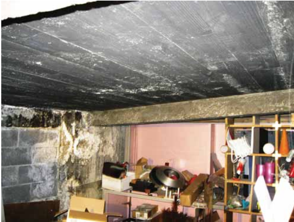
Photo 3 – Cast in place concrete area of 1 st floor at State Street entrance
