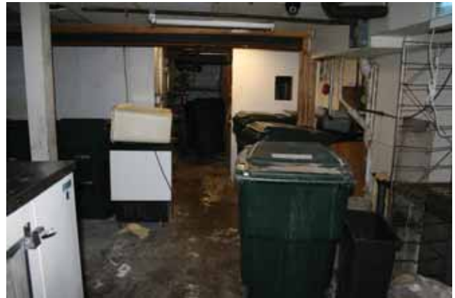
Basement: View of garbage cans
