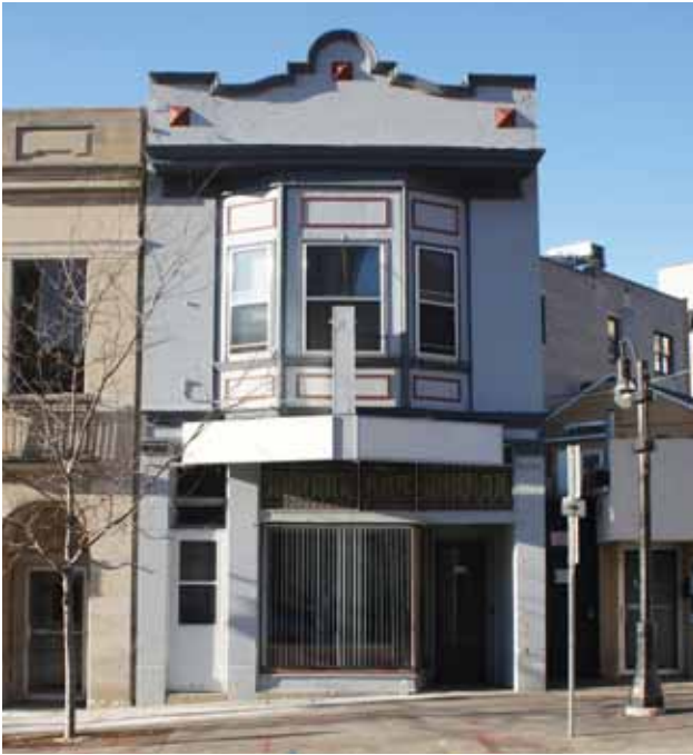
View of the Front Facade
