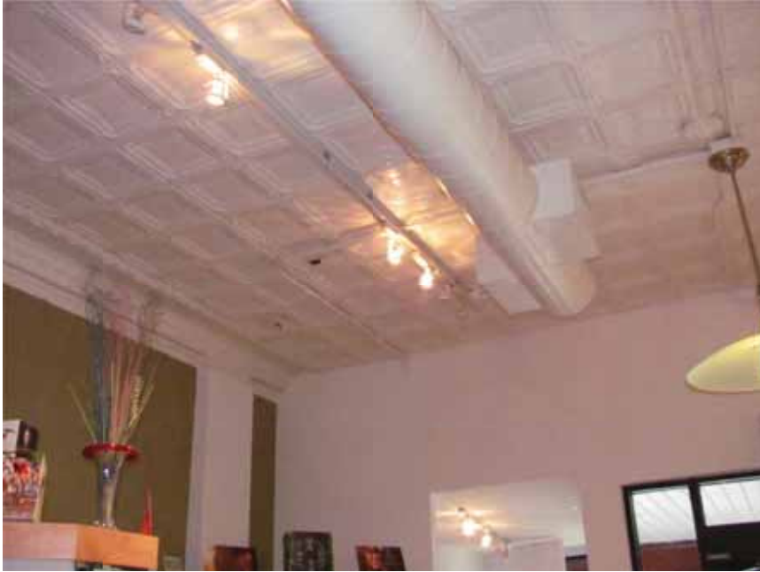
Figure 17. The ceiling in a portion of the retail space is an original painted pressed metal ceiling.
