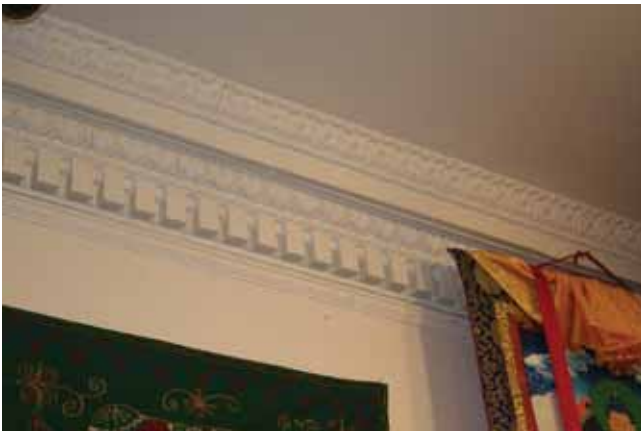
First Floor: Ceiling cornice
