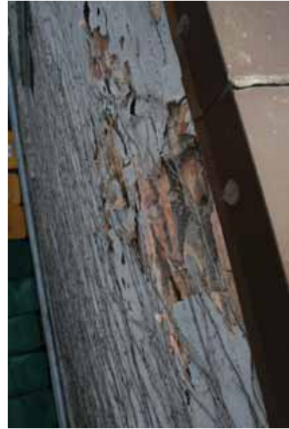
View from roof looking at condition of brick and parged wall
