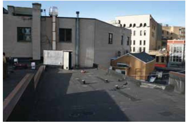
Roof showing roof access structure
