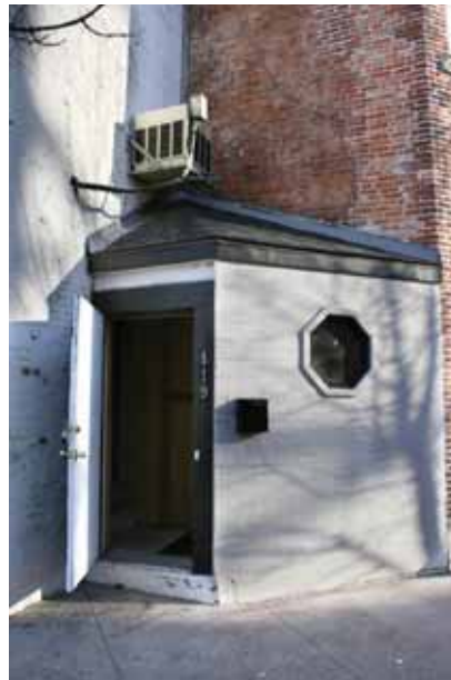
Exterior: Entry to apartment on N Fairchild Street
