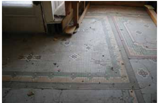
First Floor: View at entry off Mifflin Street showing three flooring surfaces. 1) Original 3/4" square tiles 2) 1" square tiles at entry 3) composite flooring at window
