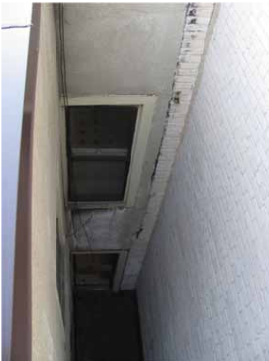
Figure 14. Two-story light well along the east wall of the building.
