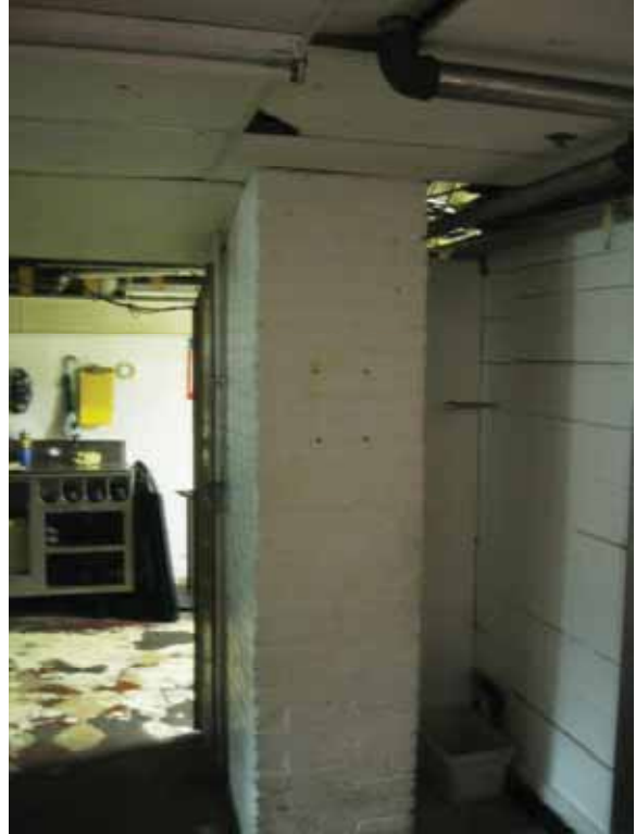
Photo 5 – Basement level brick pier
