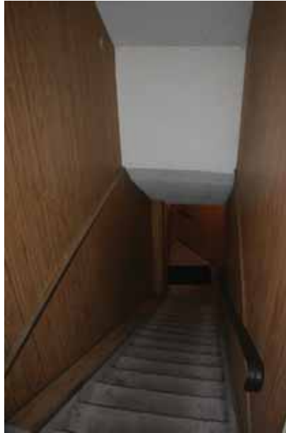
View of entrance stair access from north Fairchild Street
