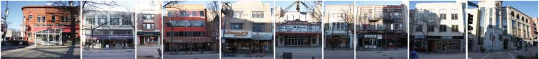
200 Block of State Street (North)
