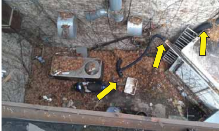
Roof drains into cistern that discharges through basement
