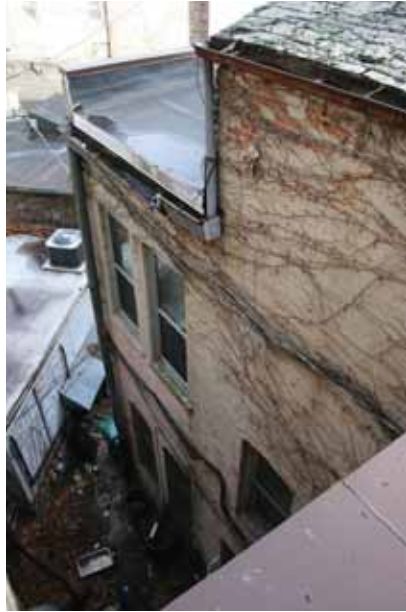
View of the back of facade
