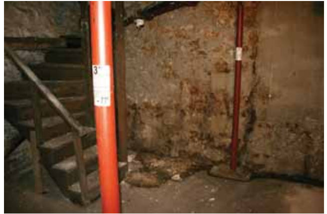
Basement: Temporary shoring to support first floor
