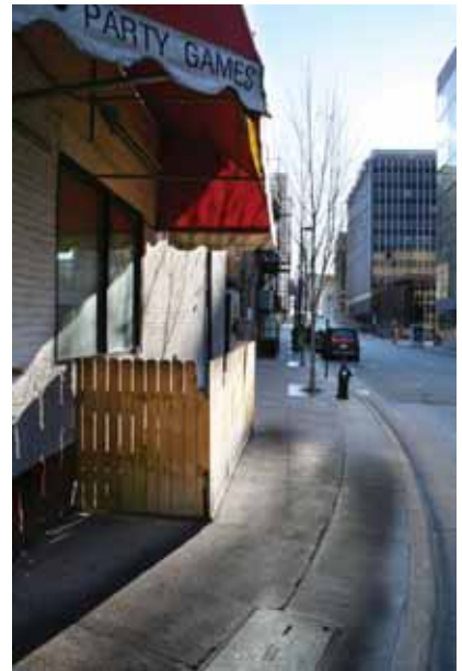
Exterior: View of basement stair access within the public right-of-way
