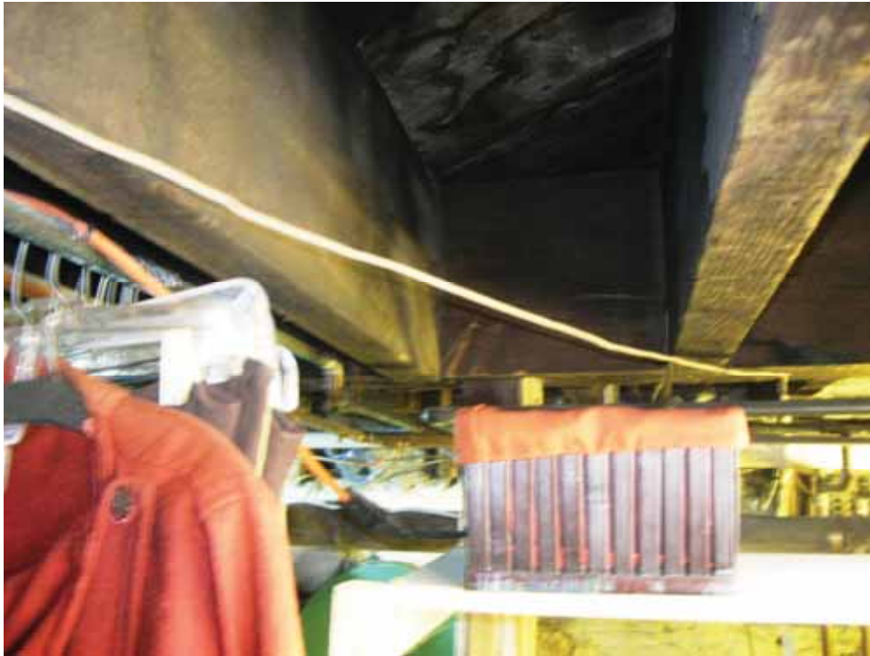
Photo 5 – 1 st floor joist framing
