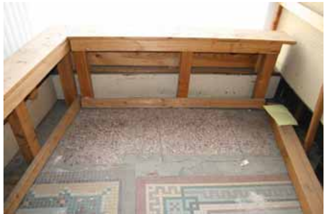
First Floor: View at bay window showing multiple types of flooring
