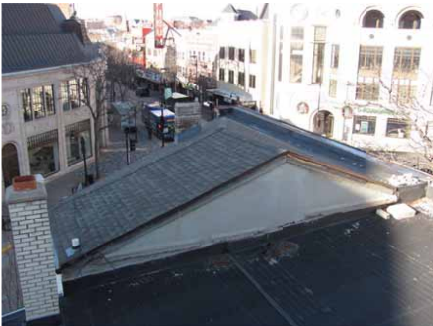
Figure 8. Overview of the roof.
