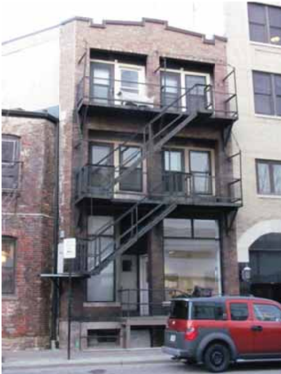
Figure 10. Overall view of the Fairchild Street facade.
