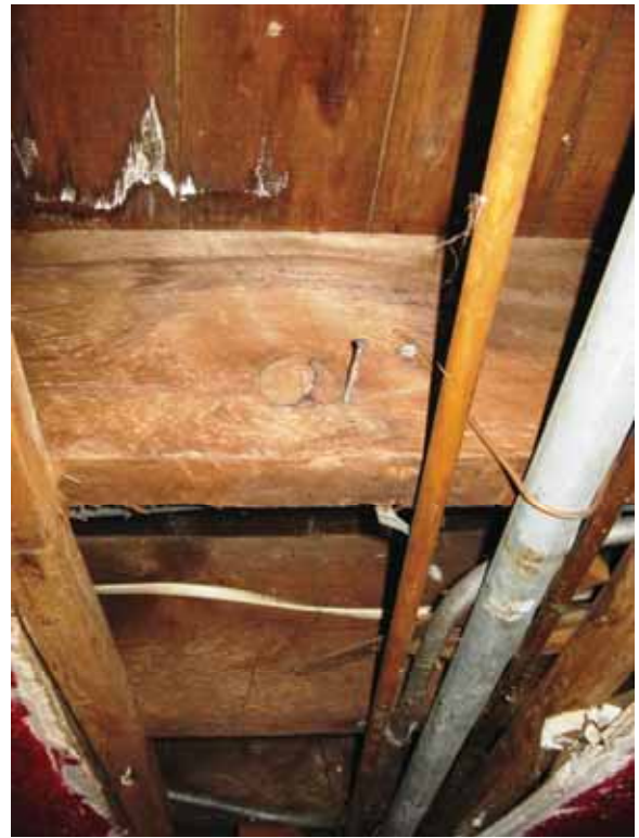
Photo 6 – 1 st floor joist framing
