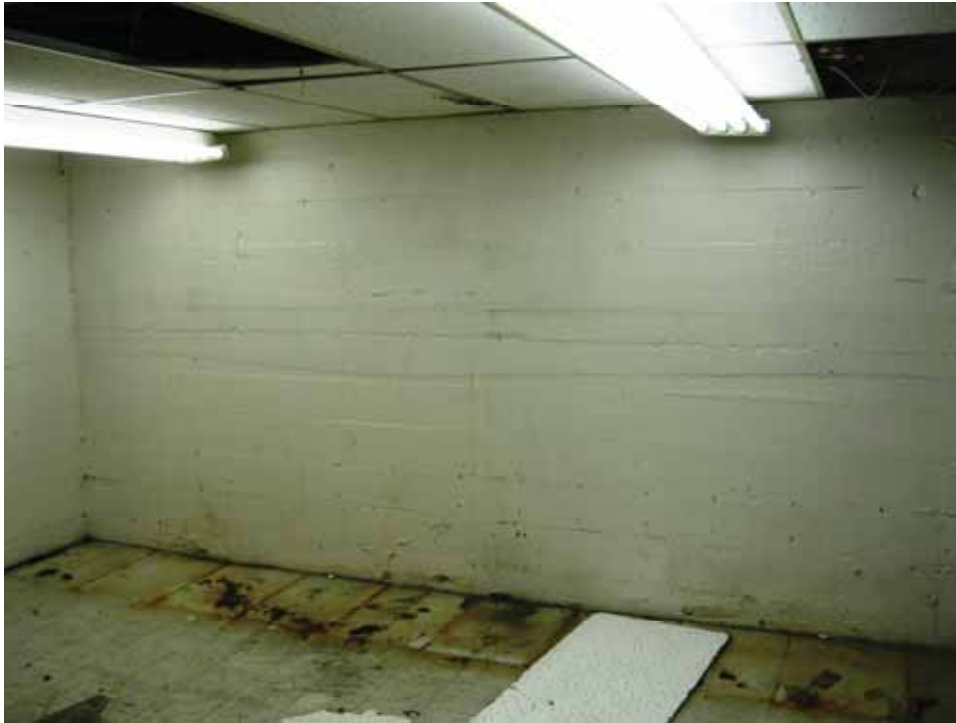
Photo 1 – Concrete basement wall at Mifflin / Fairchild corner
