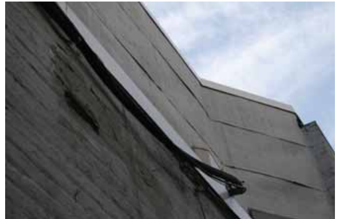
Alley view of sheet metal stamped with brick pattern
