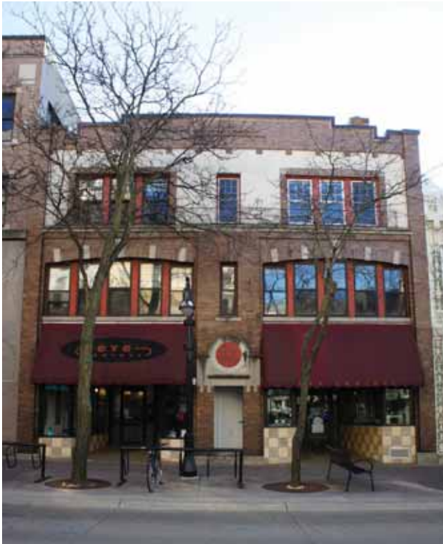
View of Front Facade
