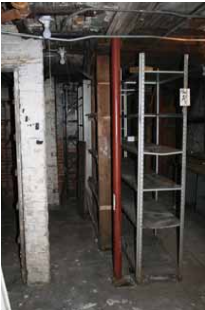
Basement: View of one temporary column supporting the first floor
