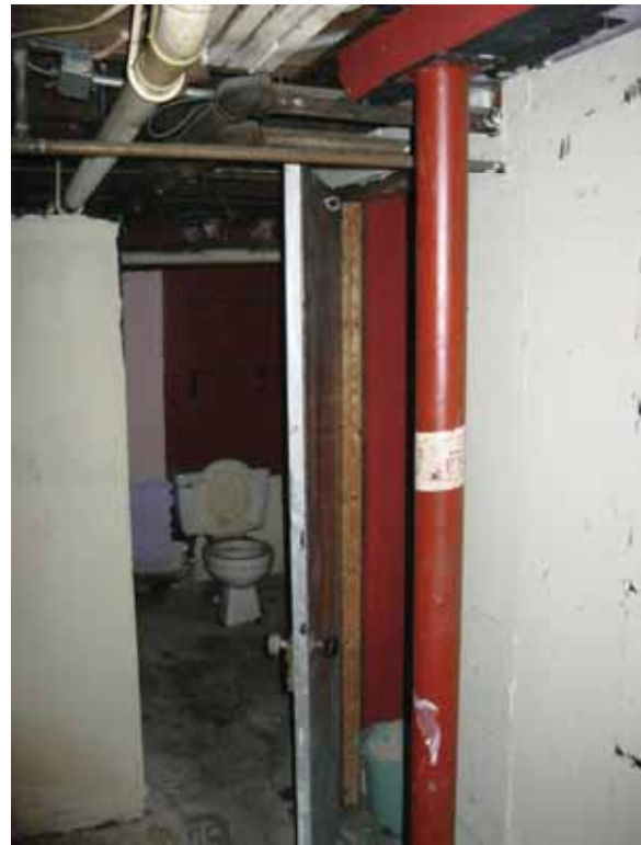
Photo 10 – 1 st floor shoring beam and post
