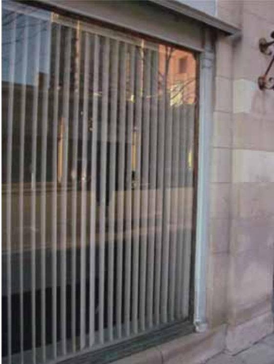
Figure 6. The storefront facing Mifflin Street has a bronze frame and fluted bronze pilasters as window jambs.
