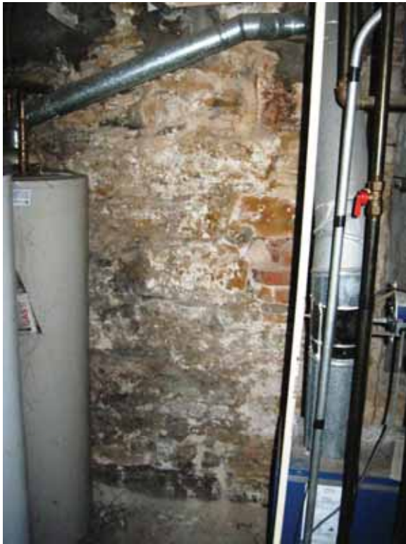
Photo 9 – Basement wall along Fairchild Street
