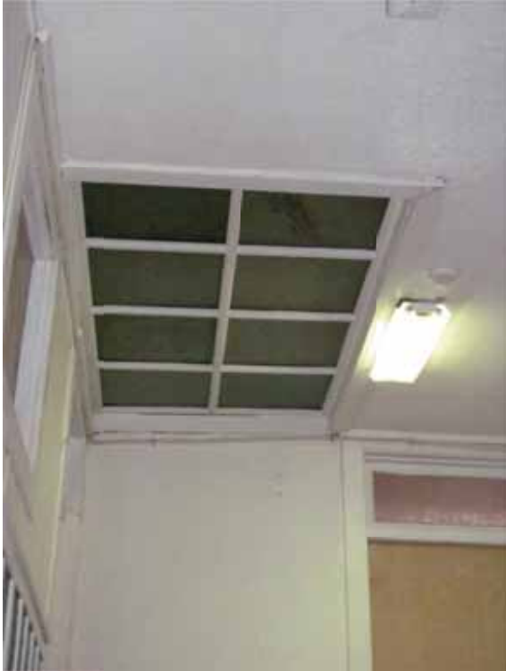
Figure 21. Interior laylight at the third floor corridor.
