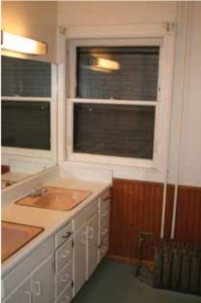
Upper Floor Apartment
