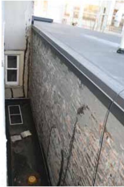
Exterior: View of side wall (party wall) between 125 state street and 121-123 State Street
