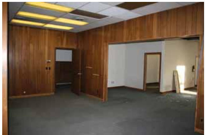
First Floor: View of office area
