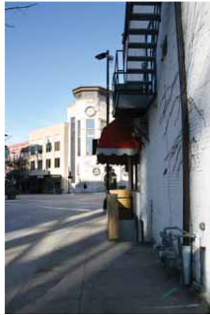
Exterior: View of basement access, gas meter and fire escape within the public right-of-way
