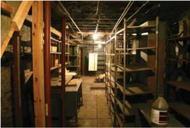
Basement: Temporary shoring to support first floor
