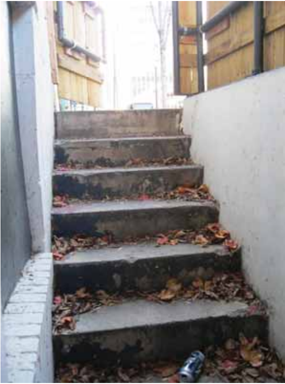
Photo 5 – Fairchild Street access to basement
