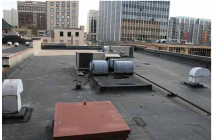
View of Roof
