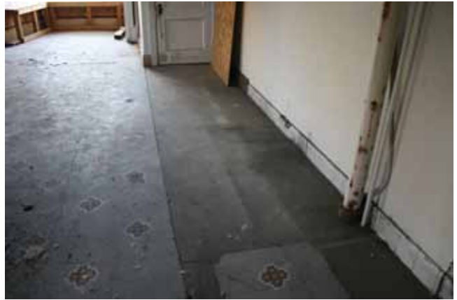
First floor: View of area where exposed concrete is installed
