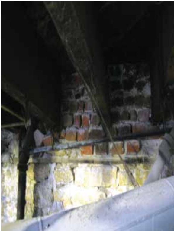
Photo 6 – 1 st floor joist bearing at basement wall 125 State Street Structural Review
