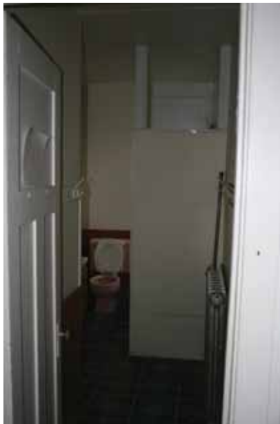
Upper Floor Apartment: Bathroom
