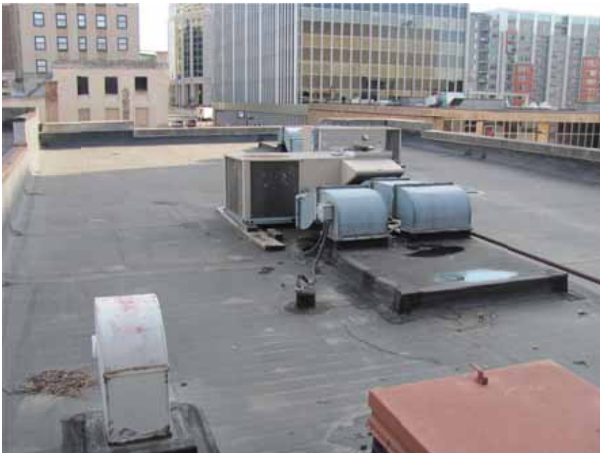
Figure 7. Overview of the roof.
