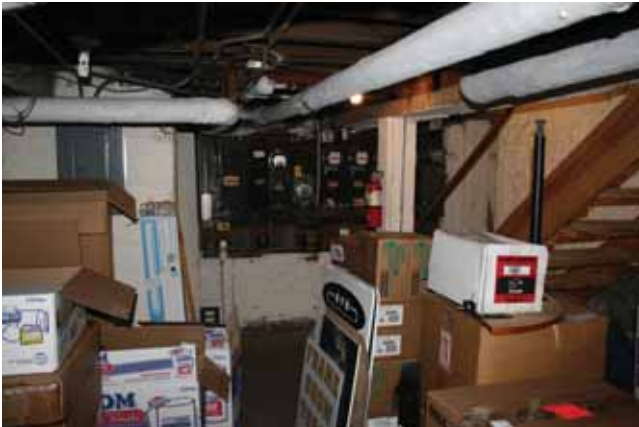
Basement: View of electrical
