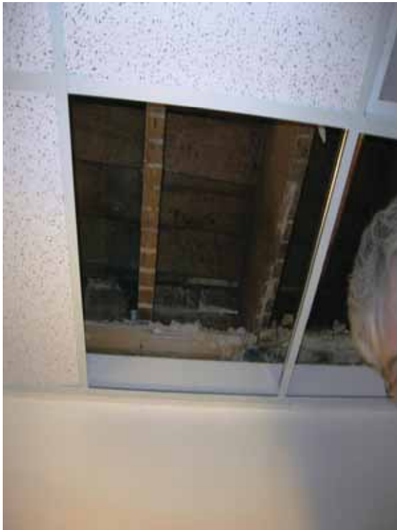
Photo 12 – 2 nd floor joist framing observed from 1 st floor retail space
