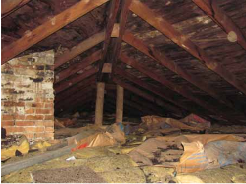
Figure 9. View of the roof framing from the attic.
