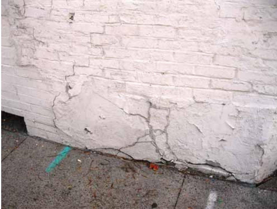
Photo 11 – Exterior wall base at Fairchild Street sidewalk
