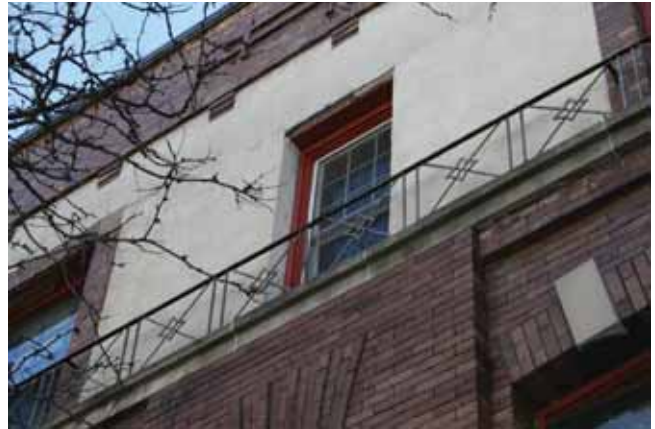
Exterior: View of plaster-coated wall surface
