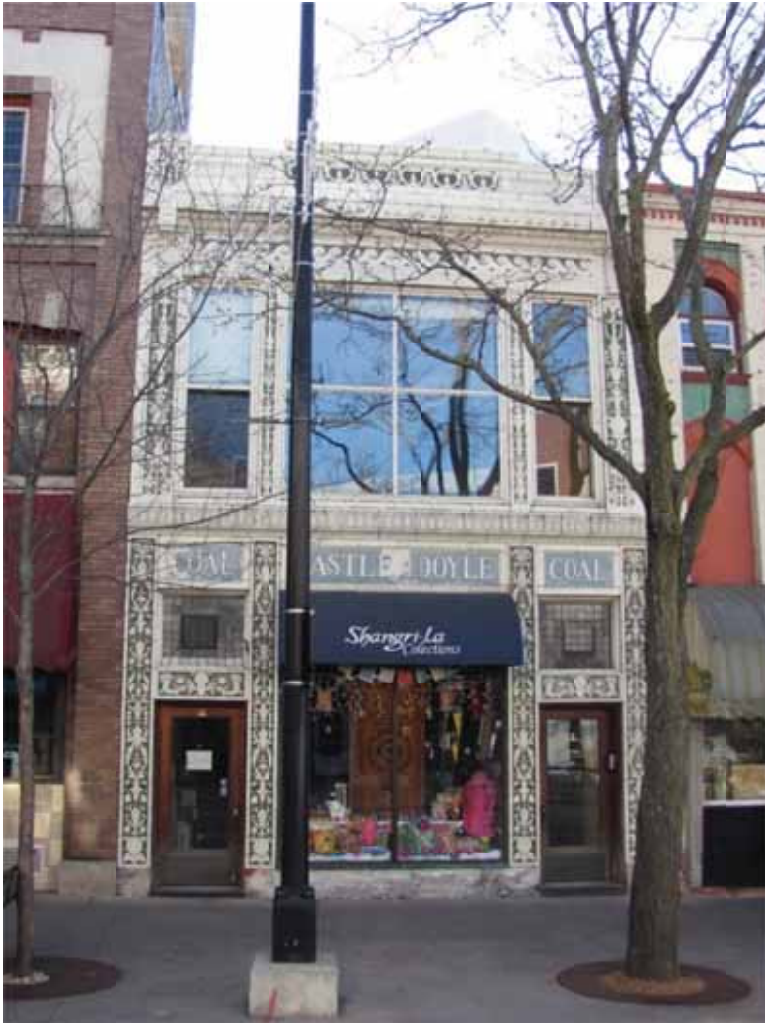
Figure 1. Overall view of the State Street facade.
