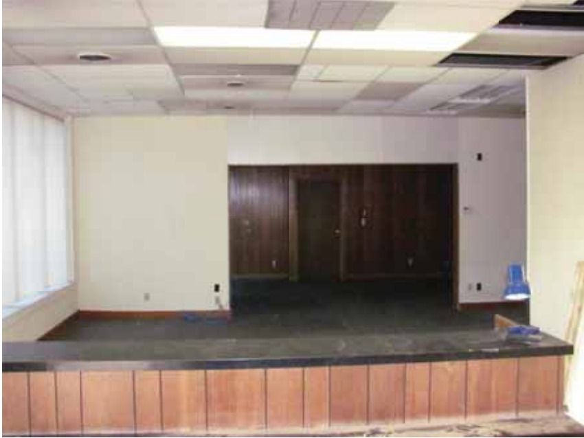
Figure 8. View of the interior.
