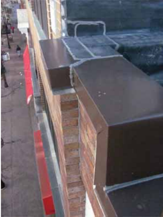
Figure 15. The sheet metal coping covers the original limestone coping.
