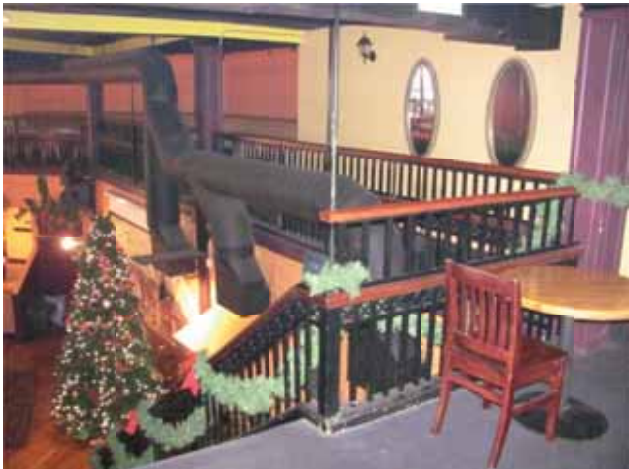
Figure 11. Second floor mezzanine with original balustrade.
