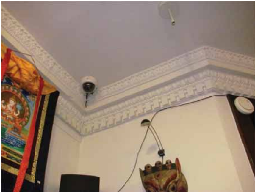
Figure 16. Plaster crown molding in the first floor retail space.
