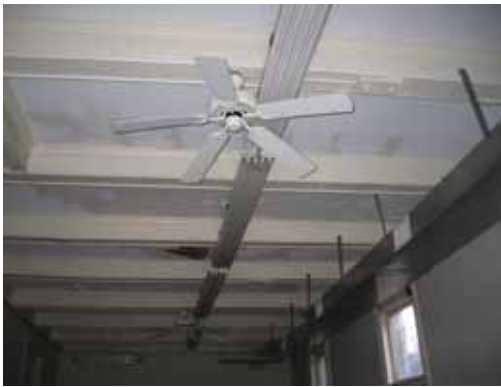
First floor lights.
