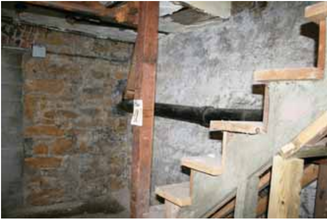
Basement: stormline routing to West Mifflin Street
