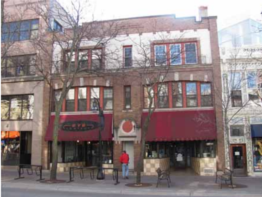
Figure 1. Overall view of the State Street facade.
