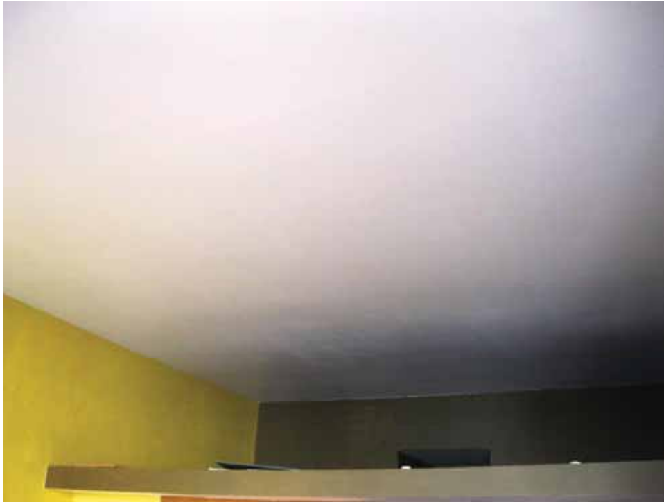
Photo 8 – 2 nd floor apartment ceiling
