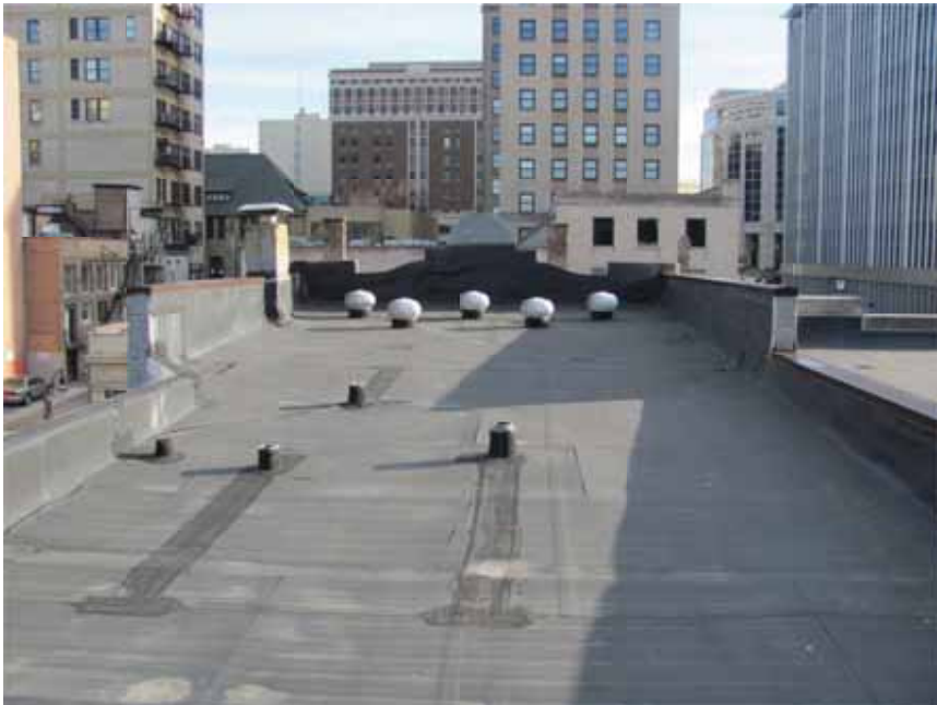
Figure 10. Overview of the roof.
