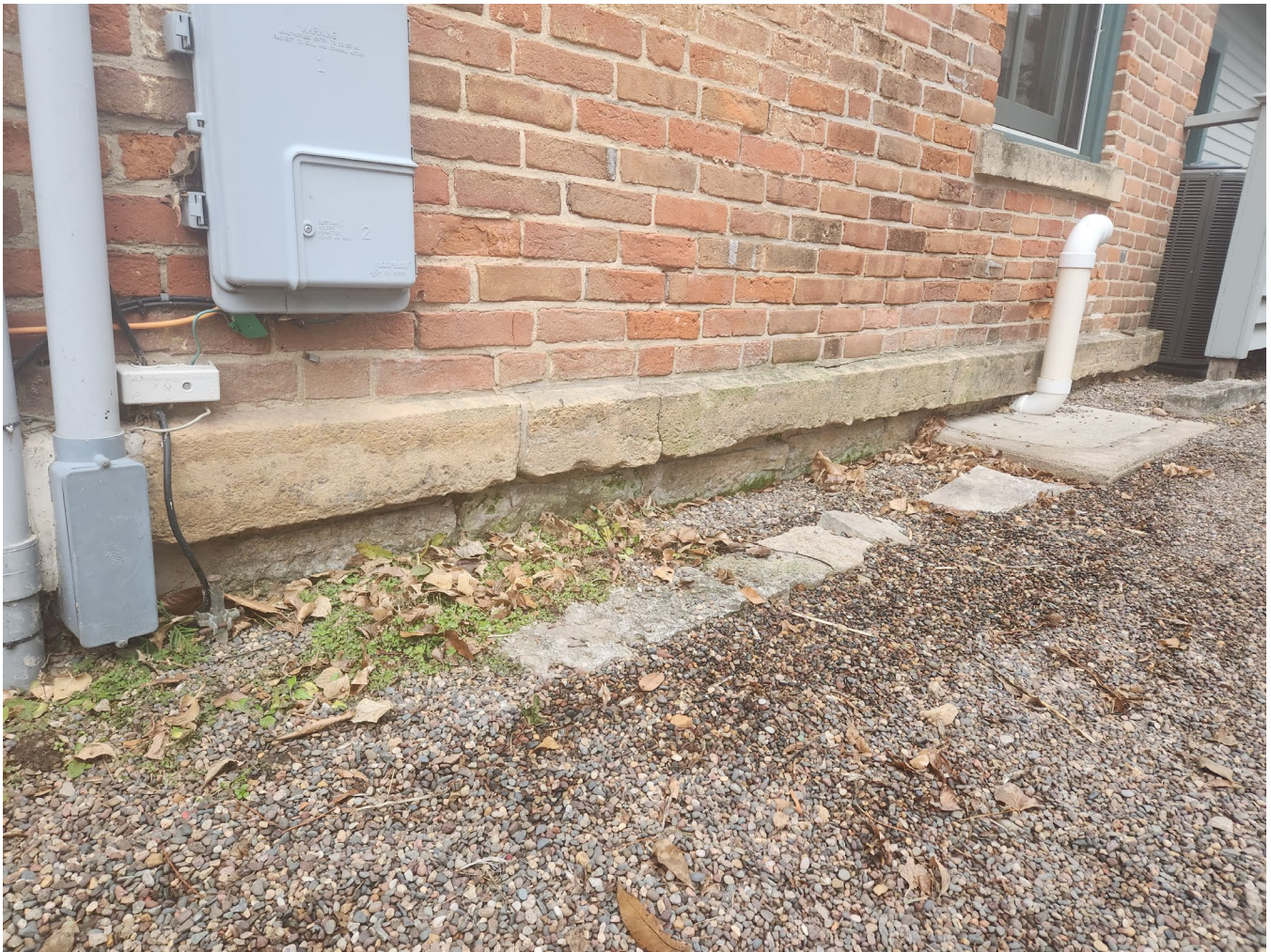
Staff photo of side of structure from 12/7/22. The limestone foundation is constructed of finely tooled, regularly coursed stone blocks, not a randomly coursed, rubble construction with untooled stone.
