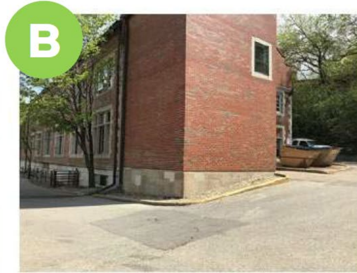
Blind corner and dumpsters at Water Science Building
