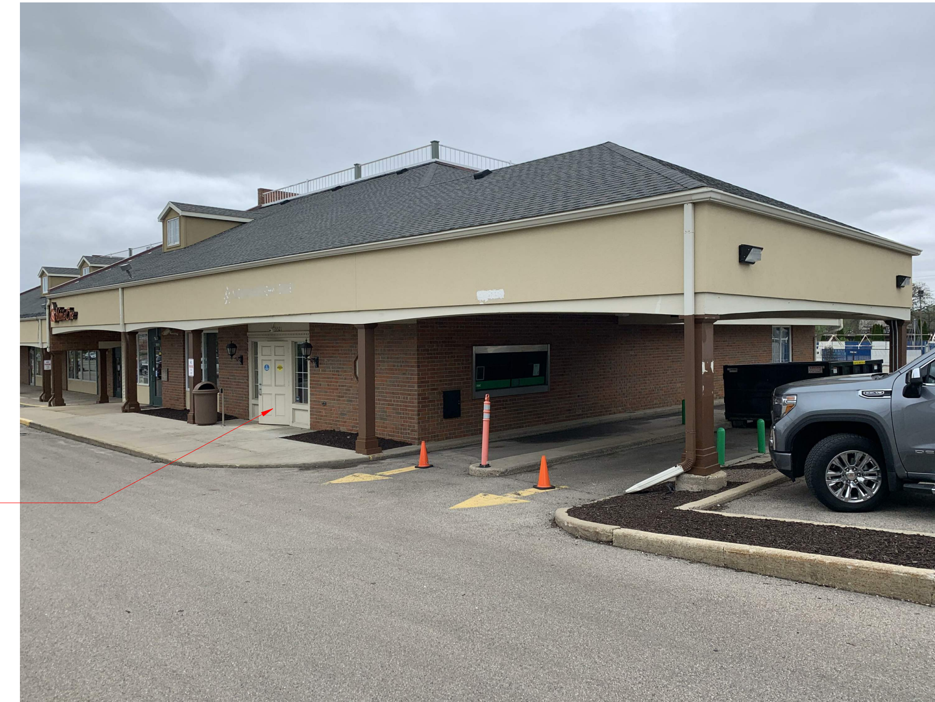
EXISTING NORTHWEST CORNER
