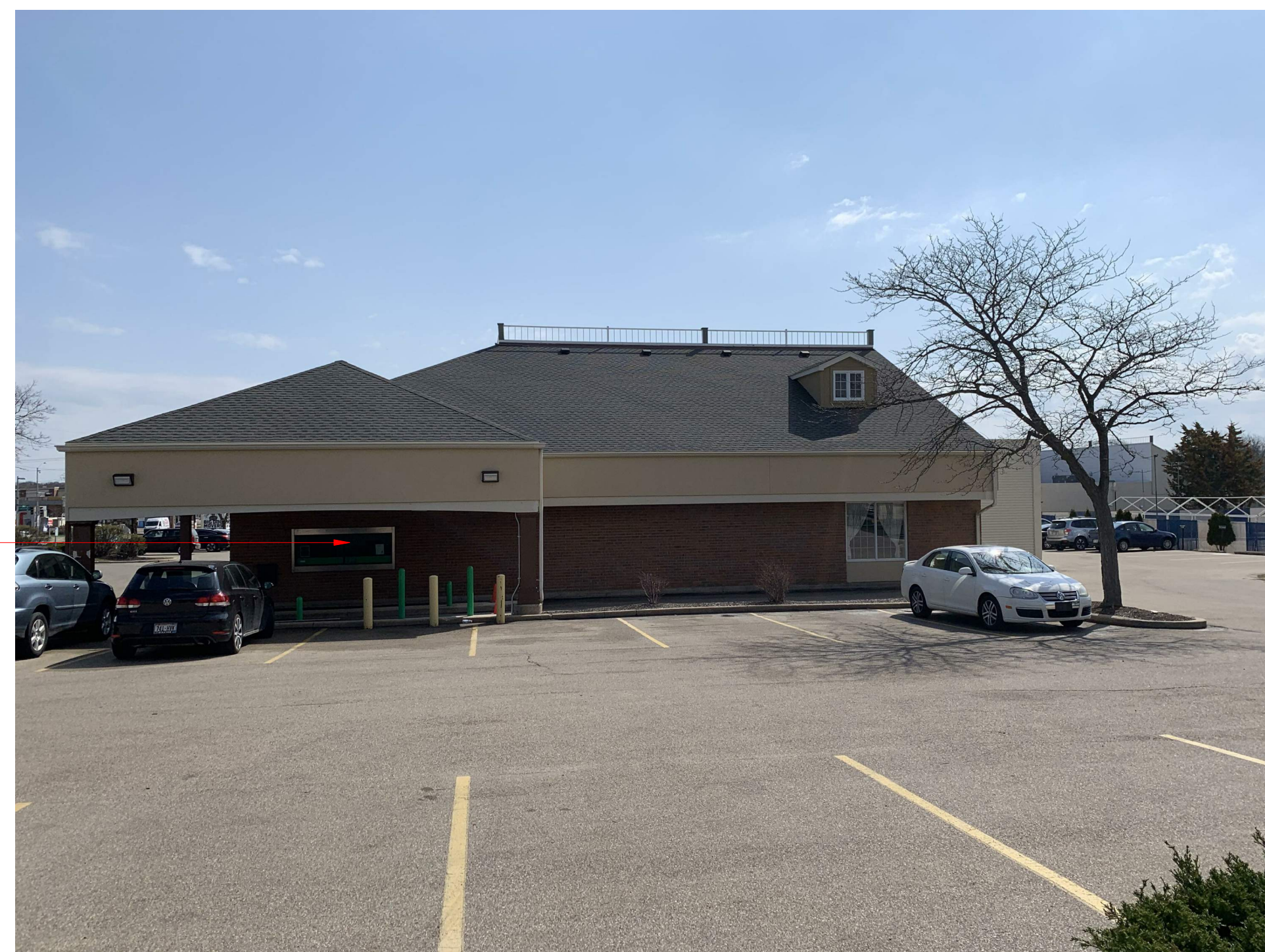
EXISTING WEST FACADE
