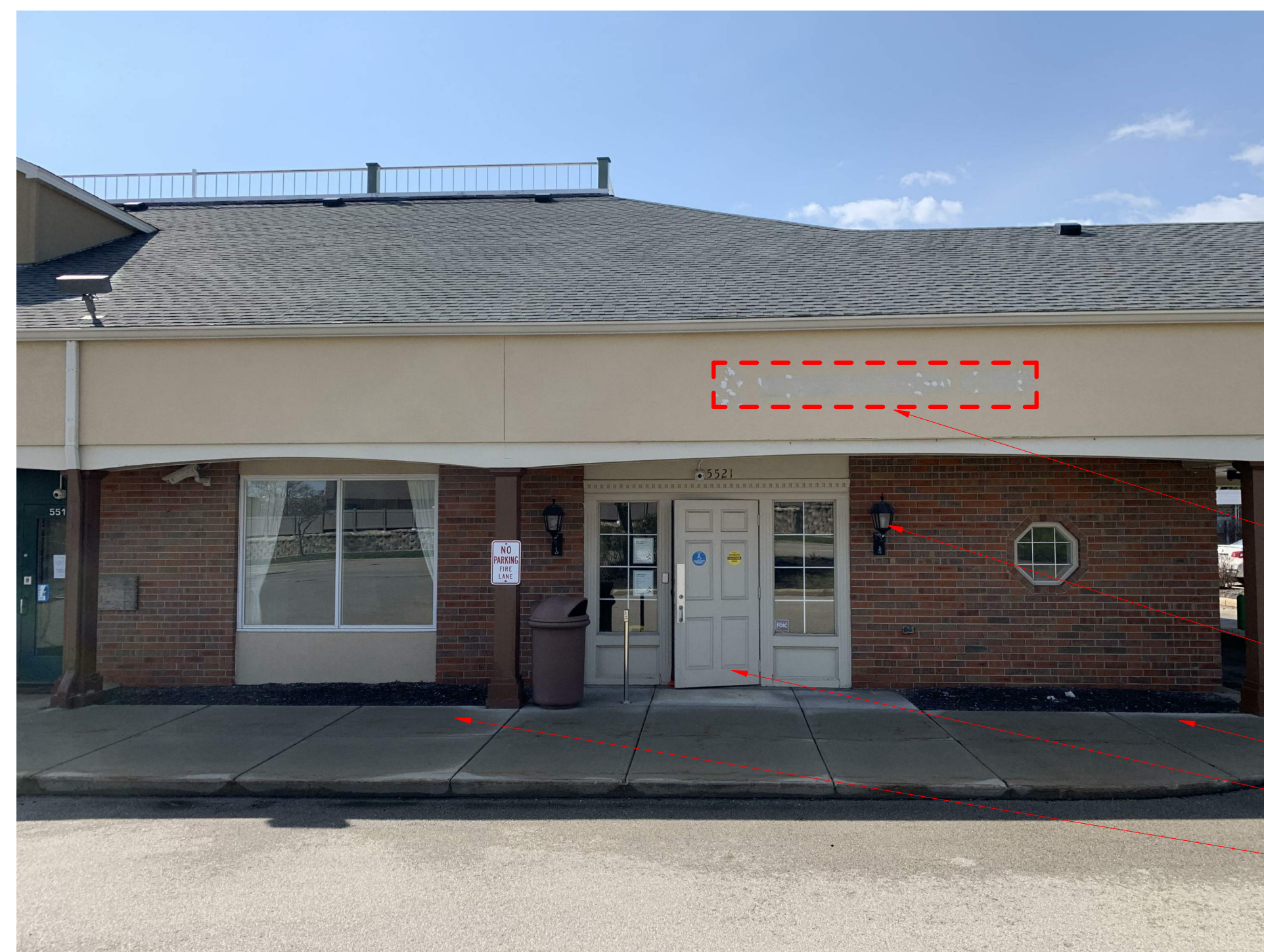
EXISTING NORTH FACADE
