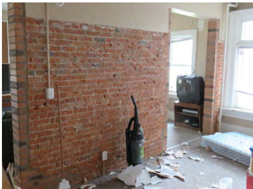
1st Floor Interior Wall
