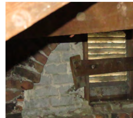
Attic, Gable end half-round window opening
