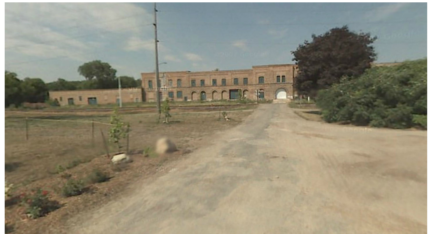
Garver Feedmill to north of railroad tracks
