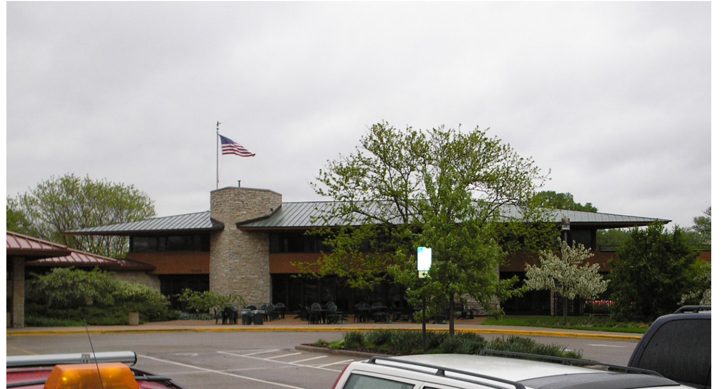
Original 1970s building
