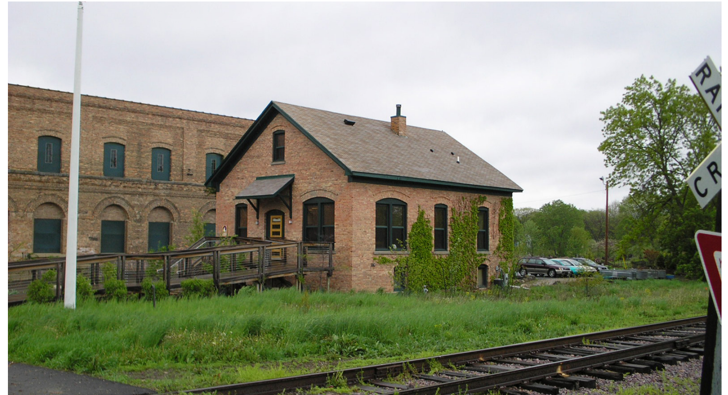
Garver Cottage (Horticulture staff office) to north of railroad tracks
