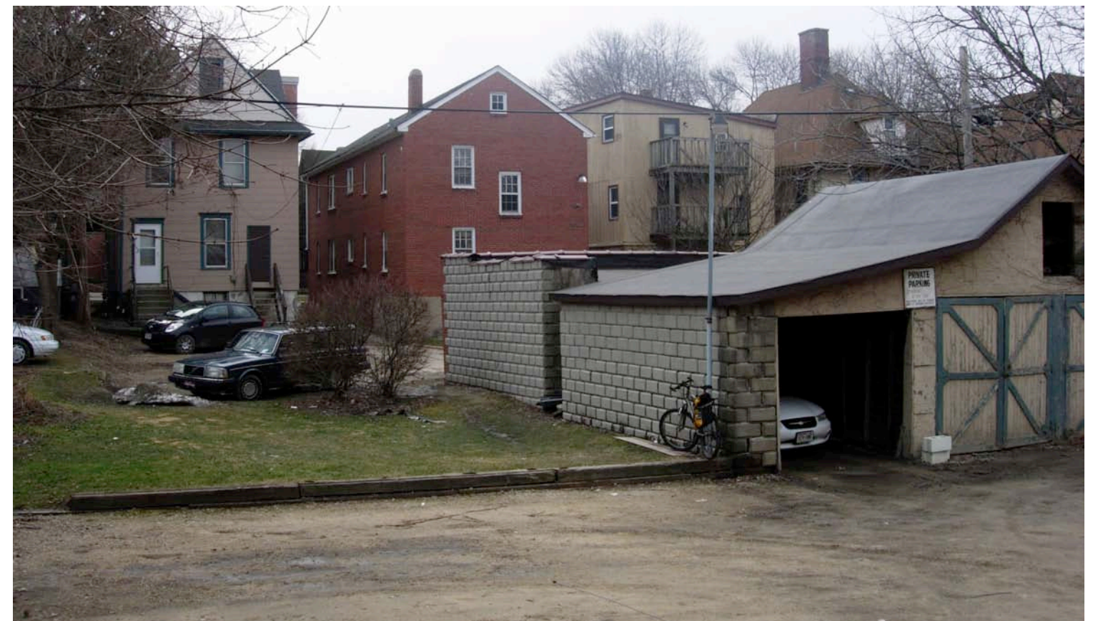
View from the South East (Rear) of 119, 123 & 125 North Butler
