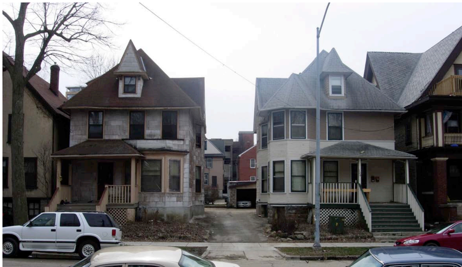
View from the East of 120 & 124 North Hancock
