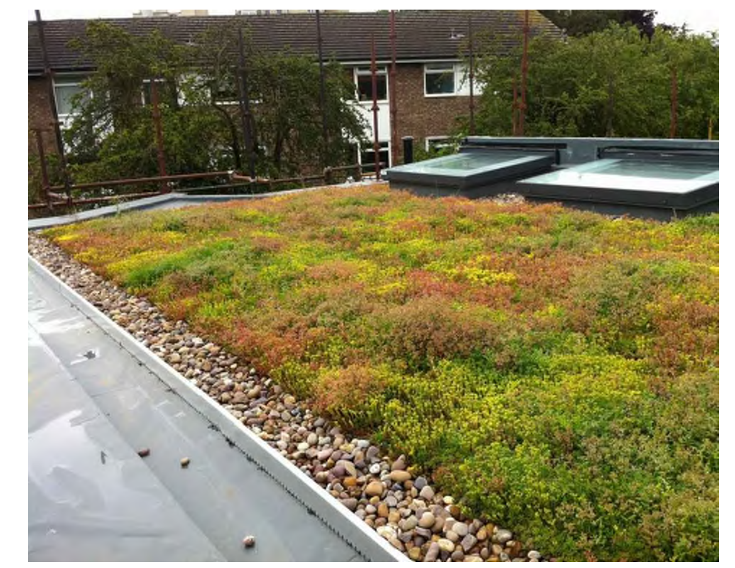
FULL SUN SEDUM CARPET GREEN ROOF WITH BALLAST EDGING - SEE PLANTING PLAN FOR MORE INFORMATION
