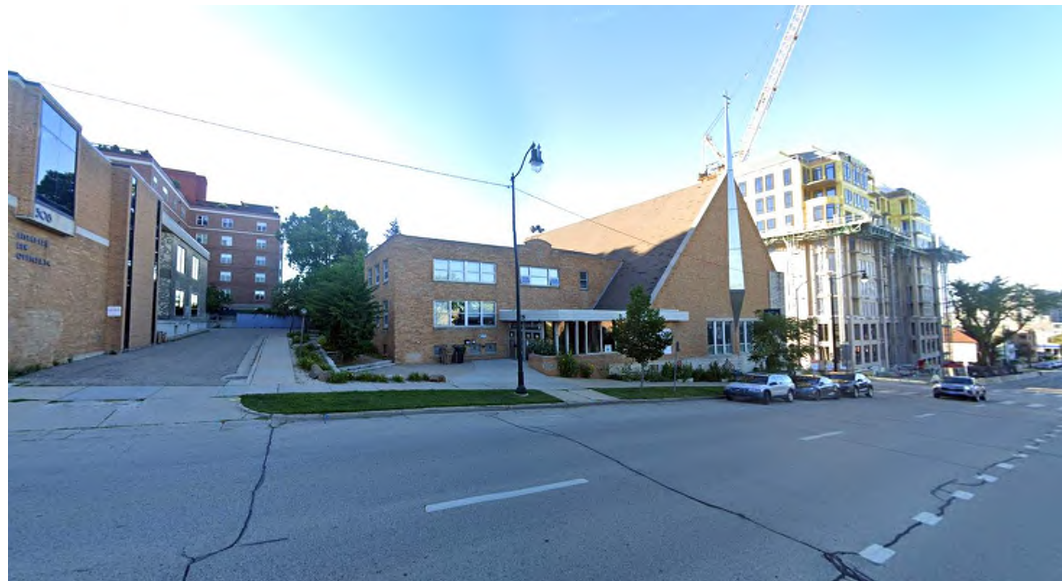
View from East Washington Avenue
