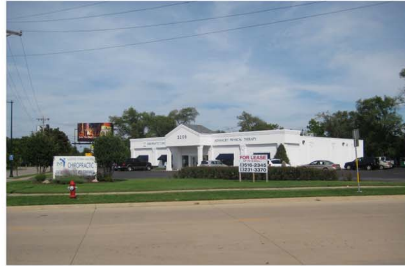
A - EXISTING COMMERCIAL BUILDING
