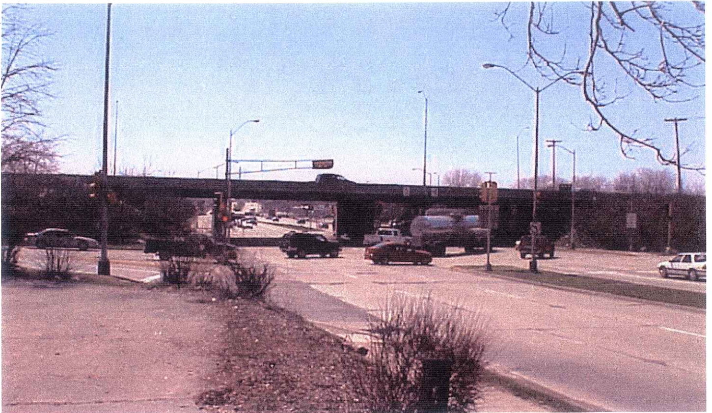
Midvale Street Frontage Facing Southwest
