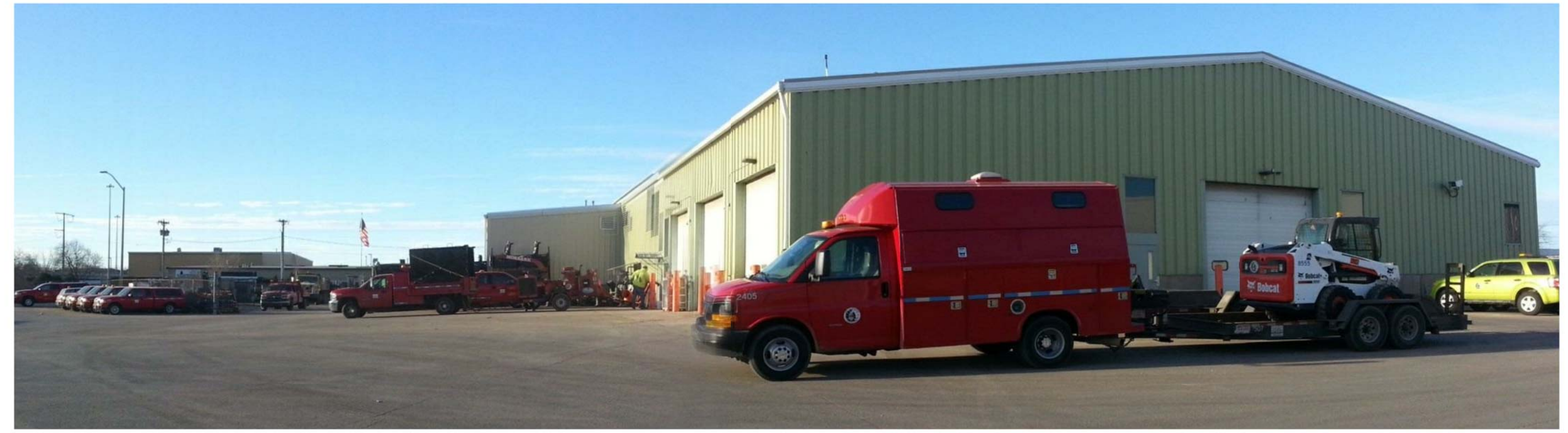
Existing View of North Elevation
