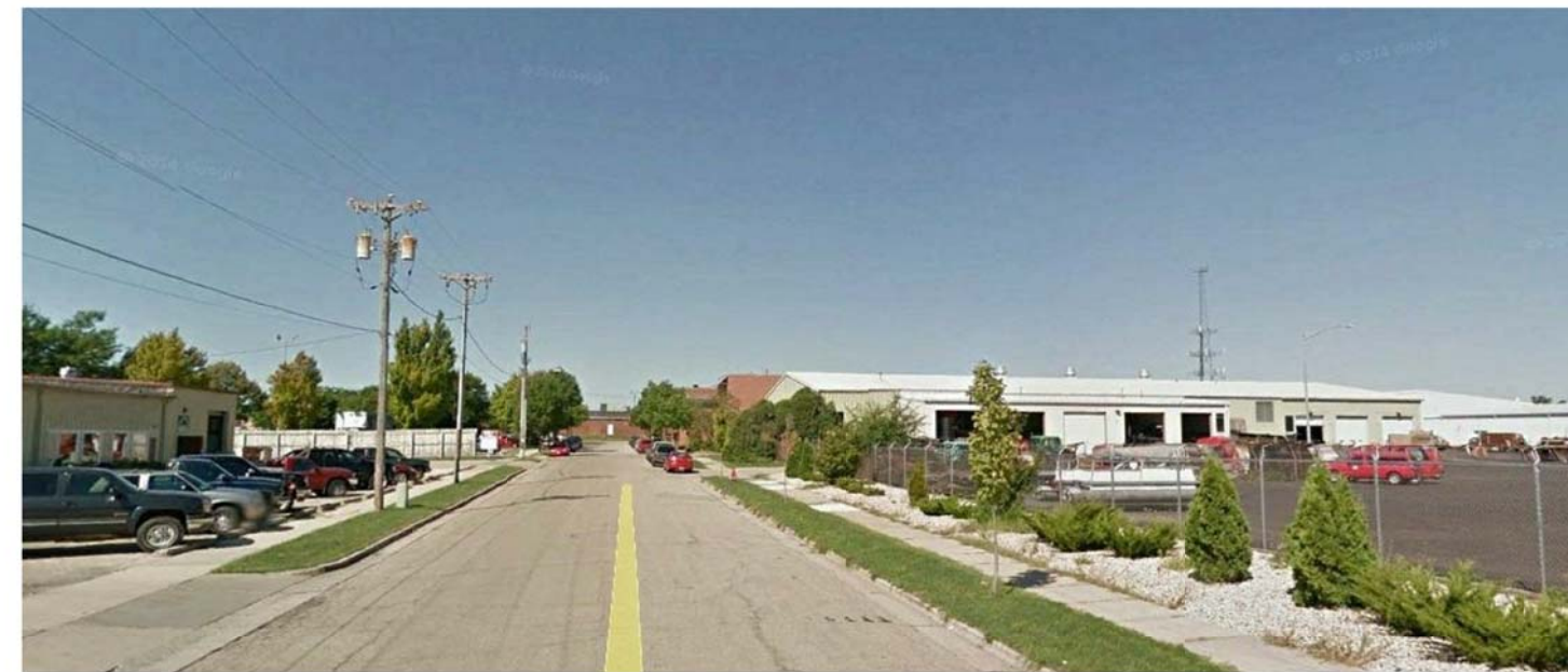
Existing View from SE
