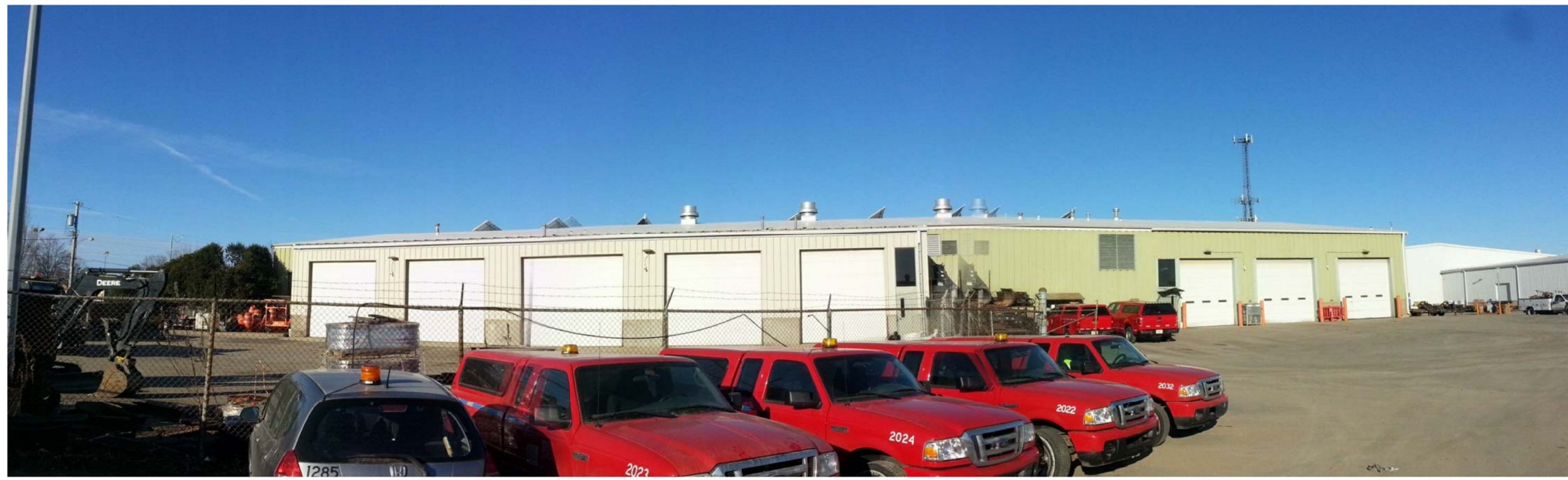
Existing View of East Elevation
