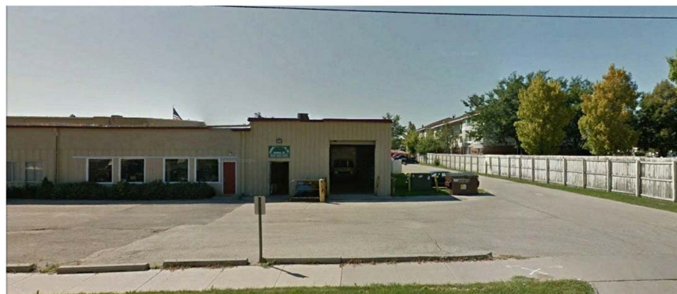
View to SE across Emil St.
