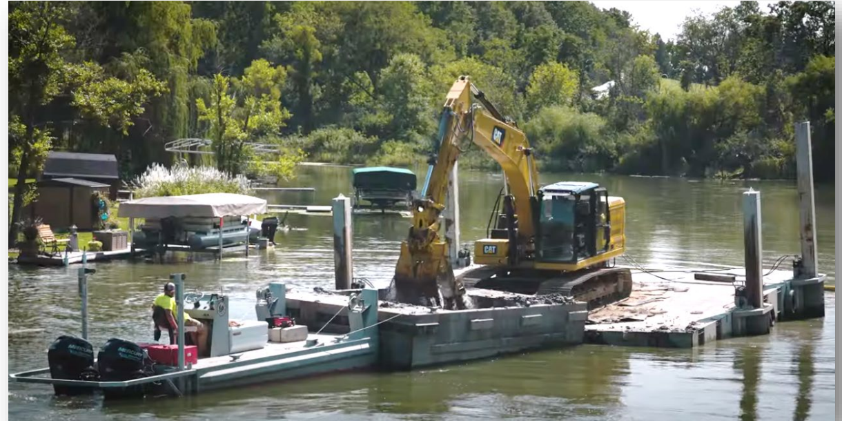
Mechanical Dredging Example
