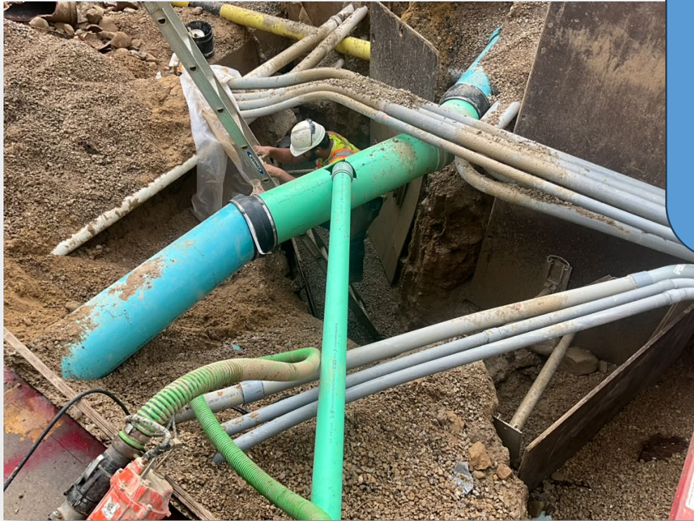
Photo: installing a sanitary sewer with Wilson St project.
