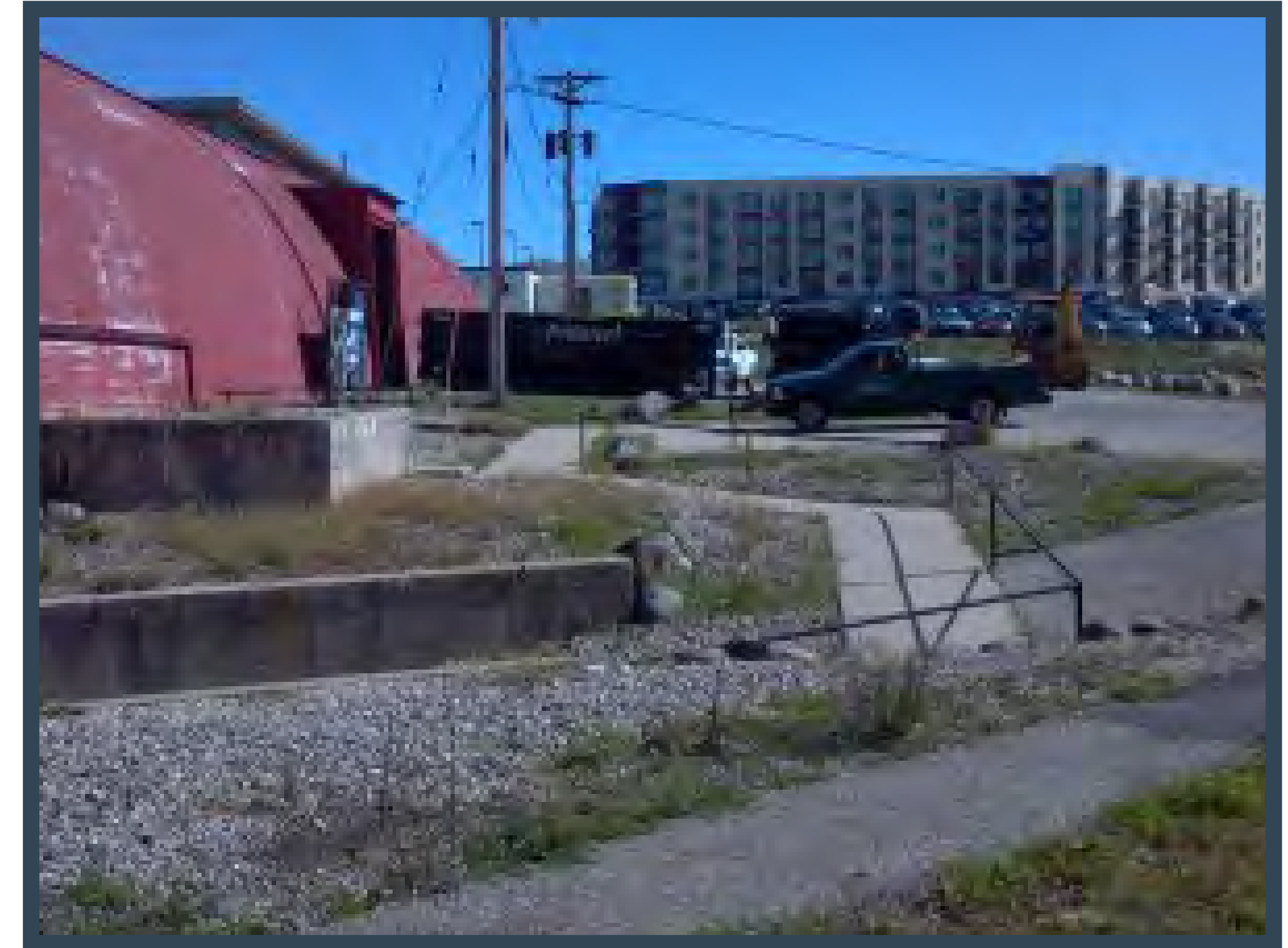
EXISTING BUILDING ON PARCEL
