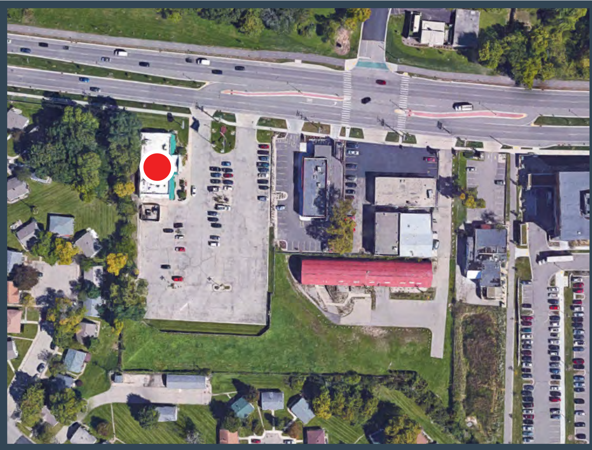
EXISTING BUILDING A (PERKINS) : LOCATION
