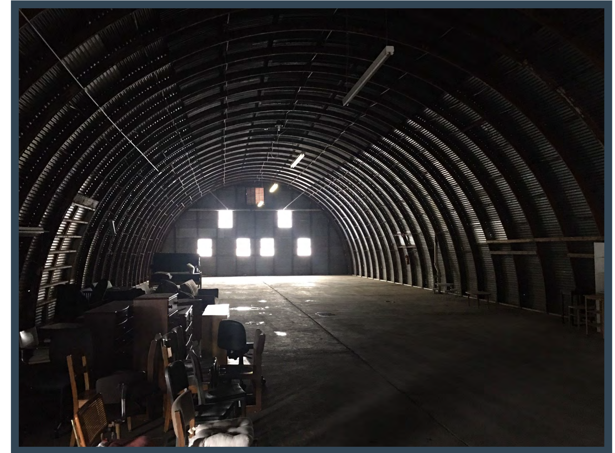
IMAGE 2 : WAREHOUSE WEST END
