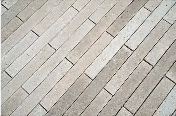
WALKING SURFACE SMALL SCALE RUNNING BOND PATTERN
