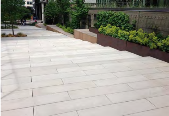
DRIVE ISLE LARGE SCALE RUNNING BOND PATTERN
