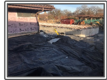
The 60,000 gallon cistern
