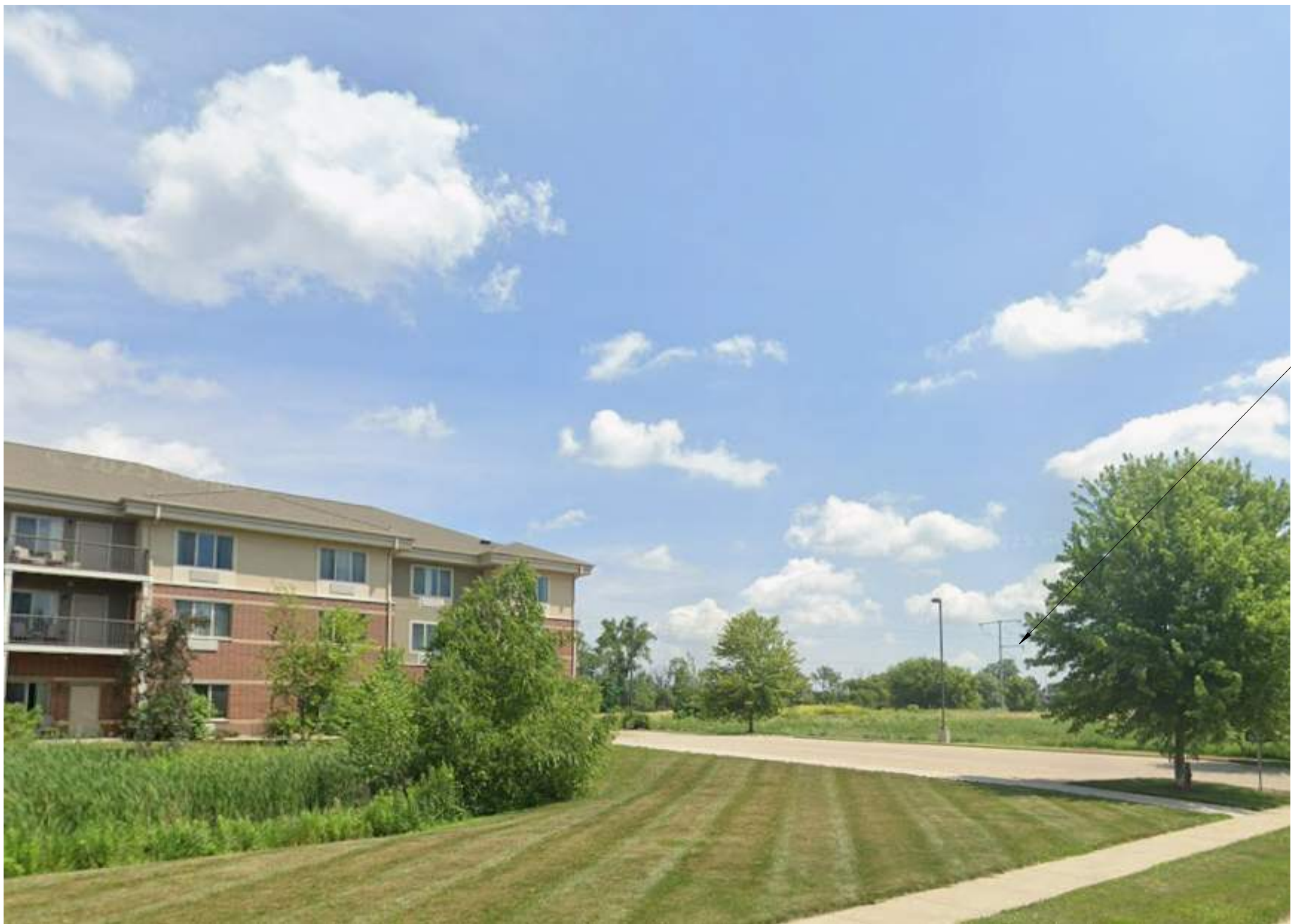
BUILDING ADJACENT TO PROPOSED BUILDING - WEST SIDE
