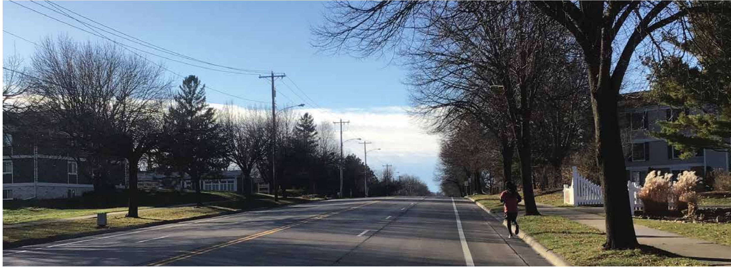
View from outside lane driving West
