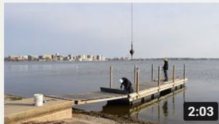
Olin Park Pier Installation
