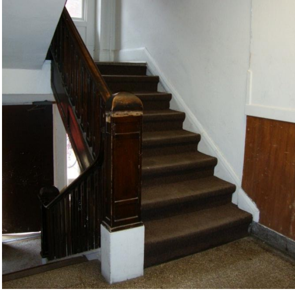
Image 1.66 View of the stairwell.
