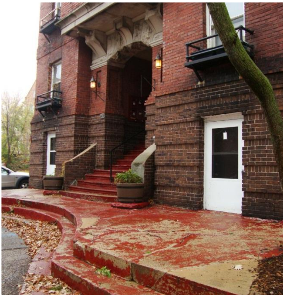
Image 1.57 North facing main entry.
