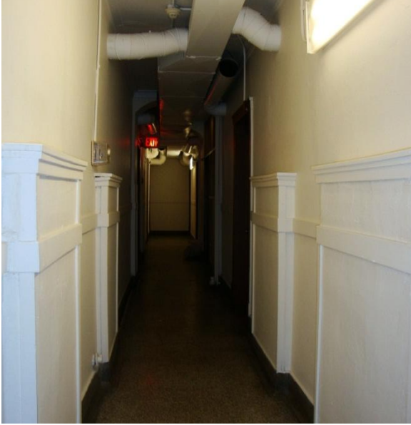
Image 1.62 View of a typical corridor.
