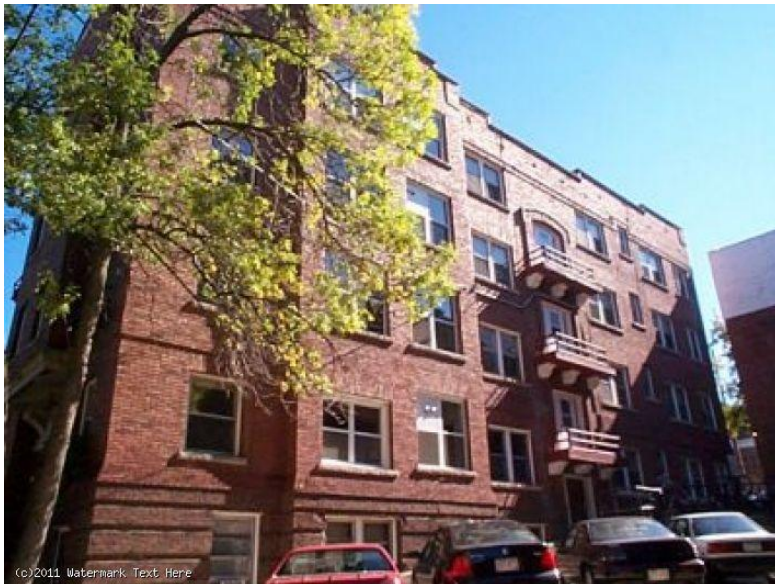
Image 1.51 View of the west elevation of 145 Iota Court.
