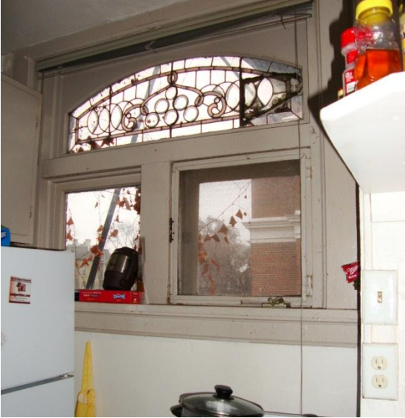
Image 1.15 View of a second floor apartment kitchen with the original tower window in the background.
