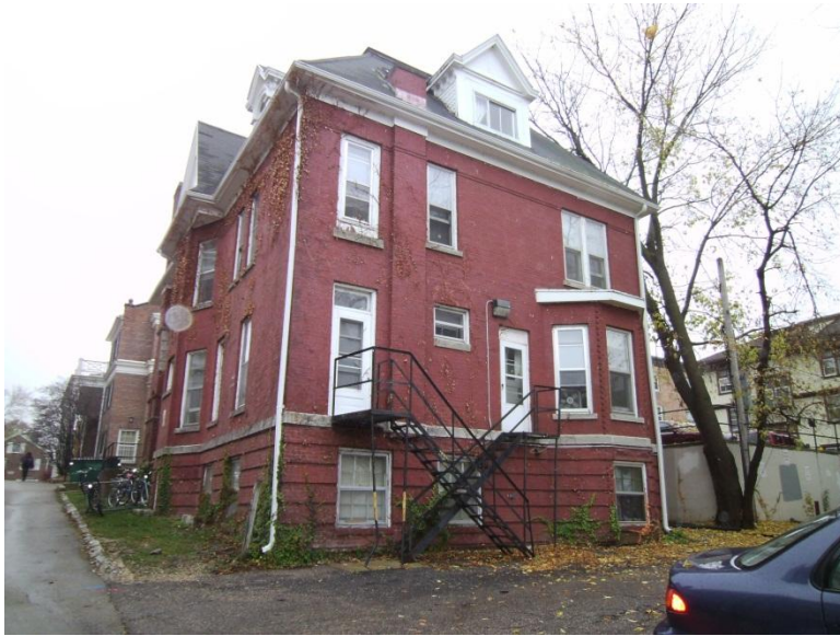
Image 1.12 View showing the north end of the building. Note the damaged columns of the fire escape.
