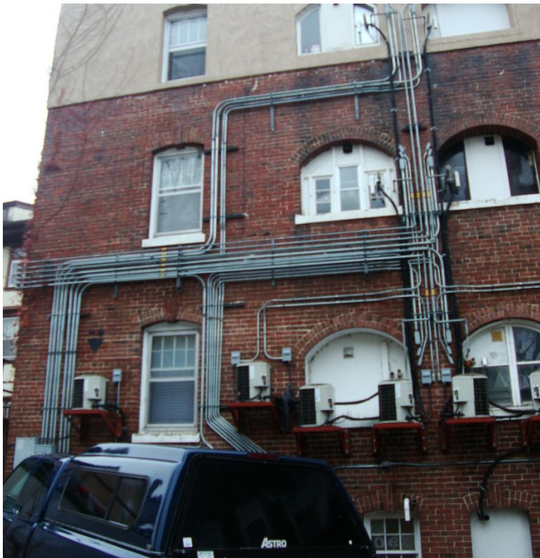
Image 1.23 View of the east elevation of the building. Note the third floor masonry has been covered with synthetic stucco. Exterior Doors and Windows
