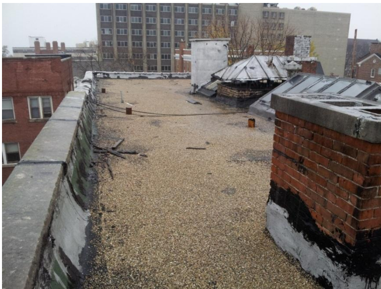
Image 1.27 General view of the roof looking west towards campus.
