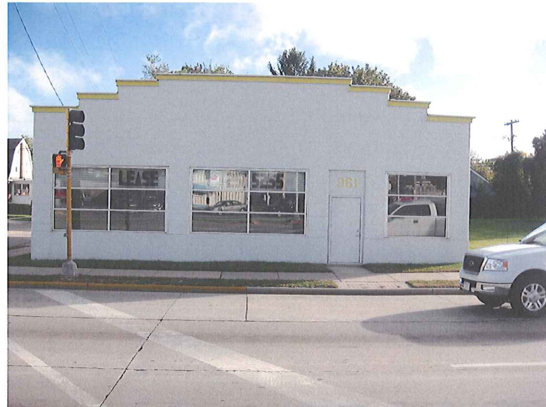
VIEW FROM PARK STREET LOOKING EAST
