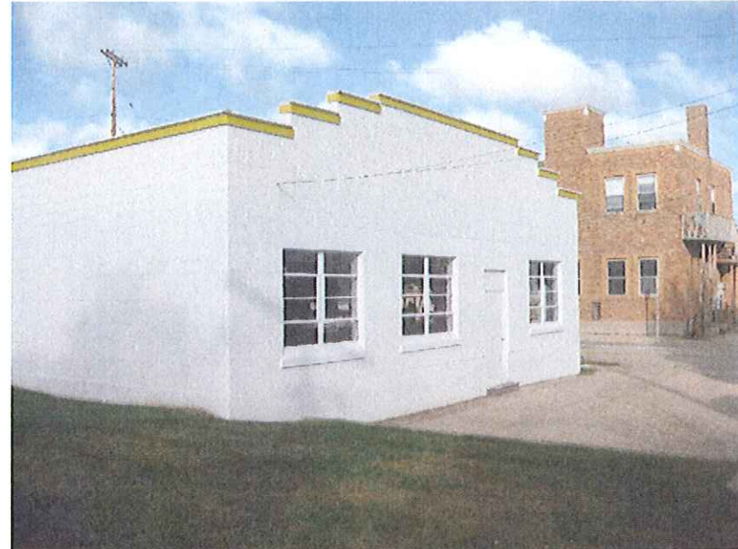
VIEW FROM 967 SOUTH PARK STREET LOOKING NORTH
