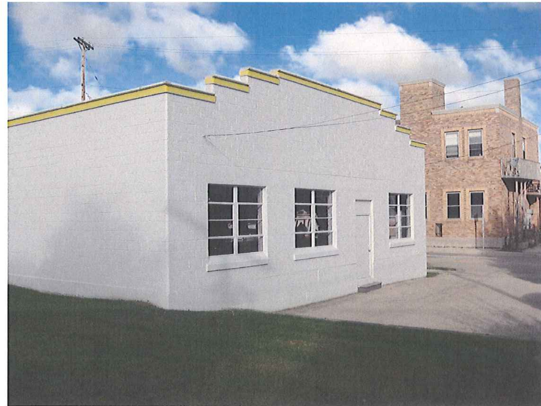
VIEW FROM 967 SOUTH PARK STREET LOOKING NORTH
