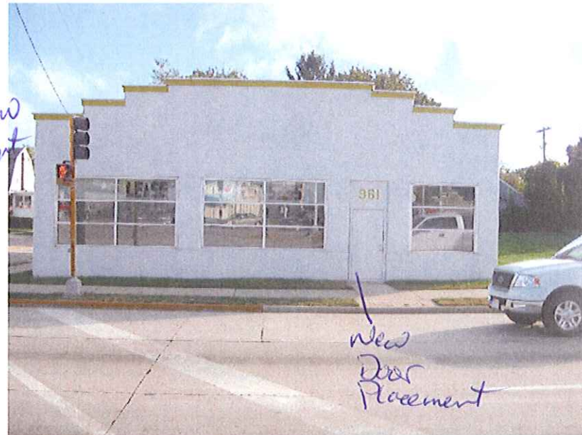
VIEW FROM PARK STREET LOOKING EAST
