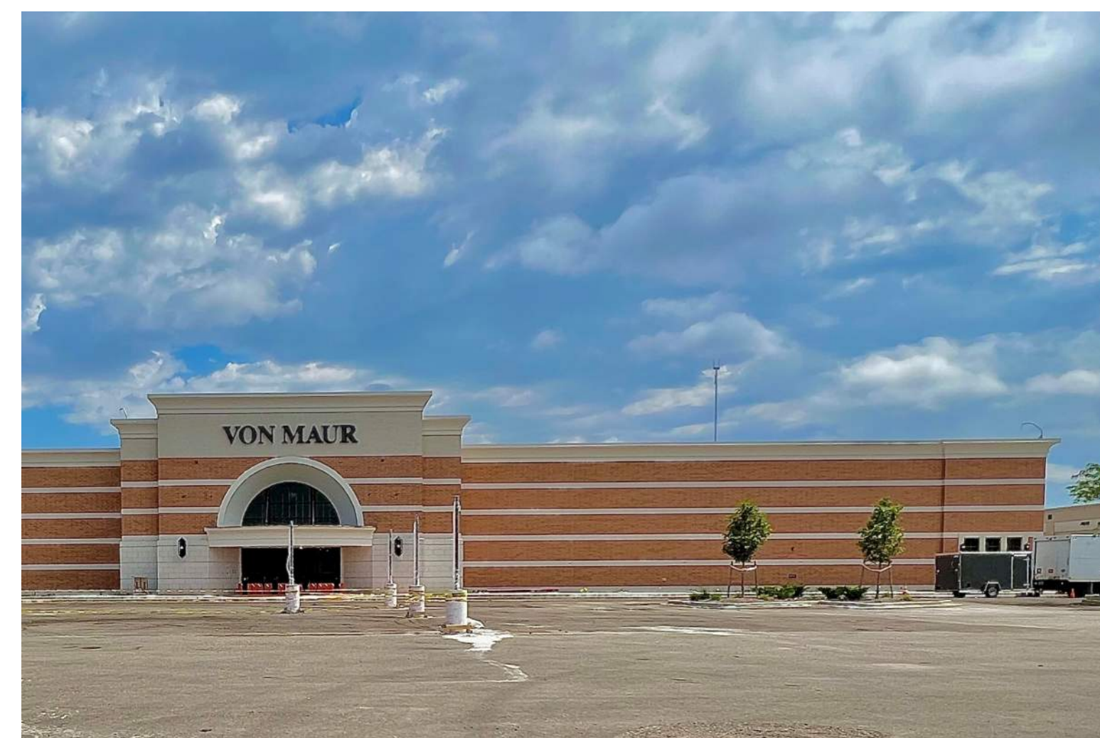
VON MAUR WEST EXTERIOR WALL
