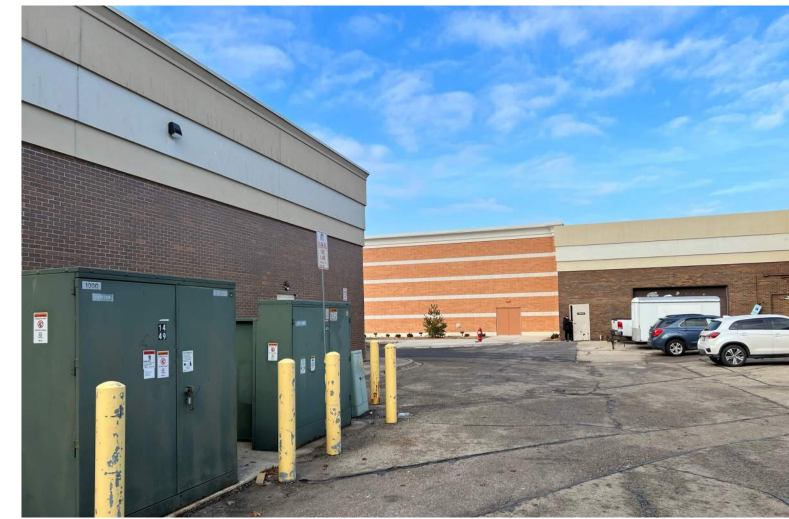
PLANET FITNESS EAST EXTERIOR WALL LOOKING TOWARD VON MAUR
