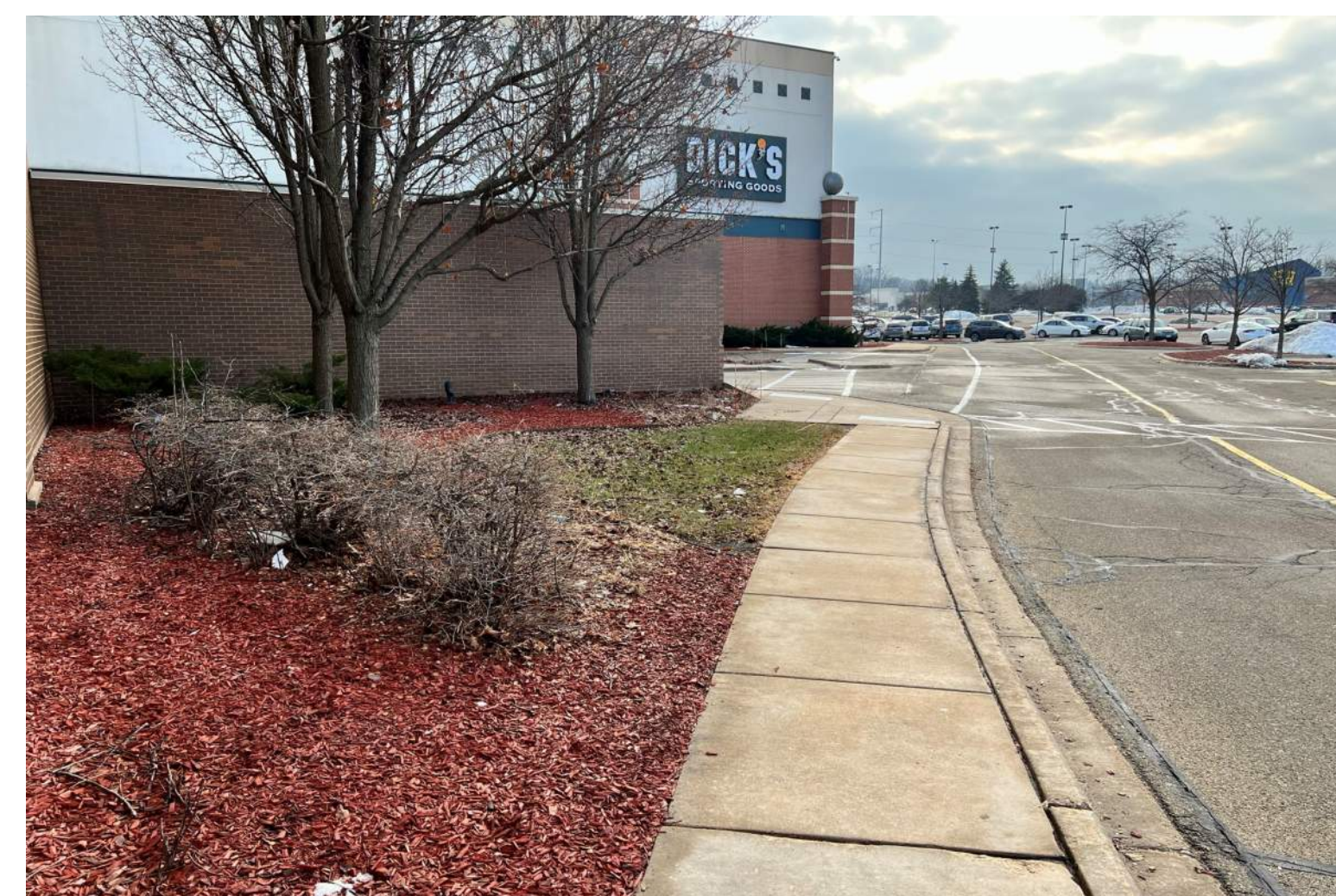
DICK'S SPORTING GOODS NORTH EXTERIOR WALL
