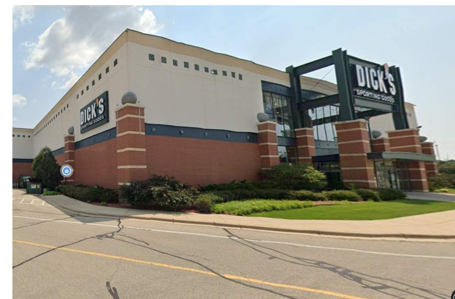
DICK'S SPORTING GOODS NORTH AND WEST EXTERIOR WALLS
