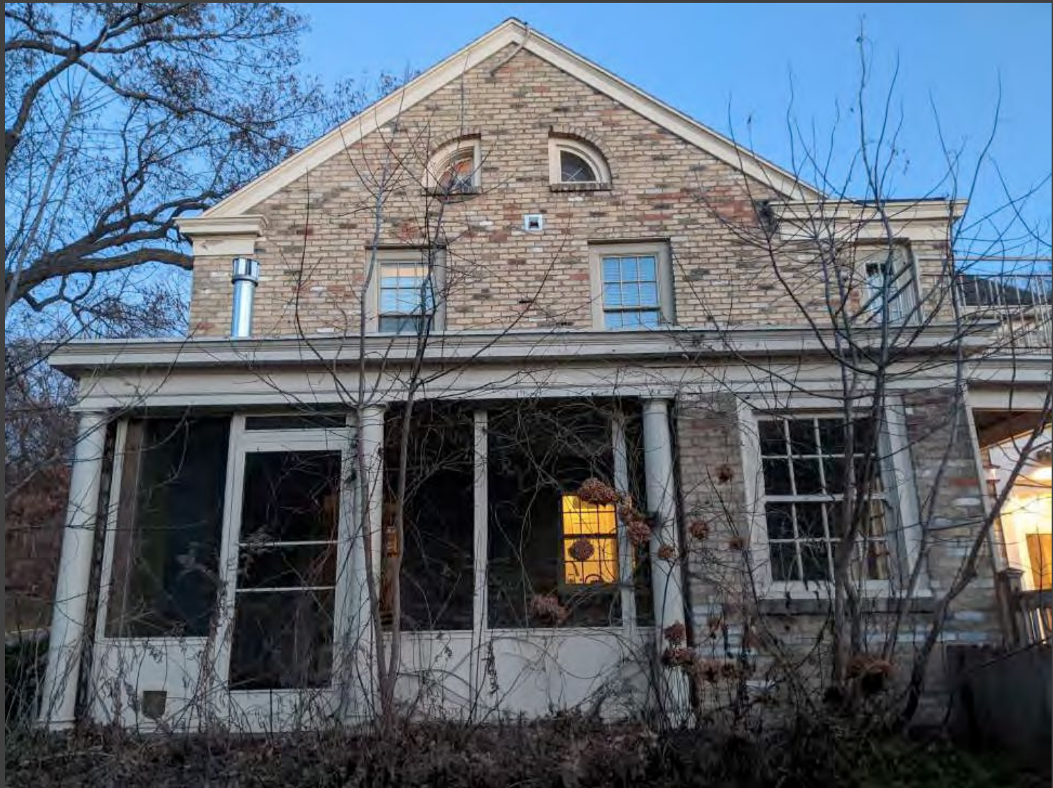
Existing site photos
