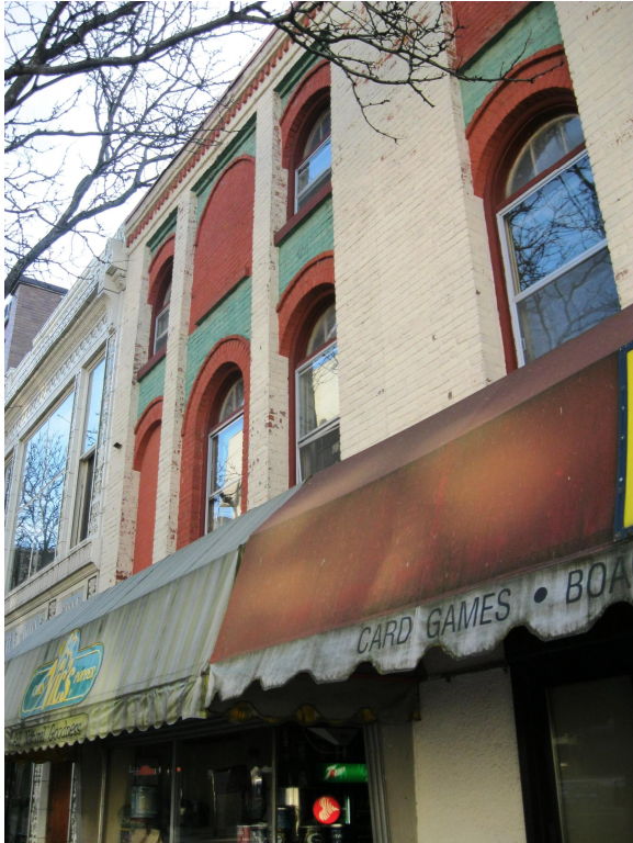
Photo 1 – State Street elevation
