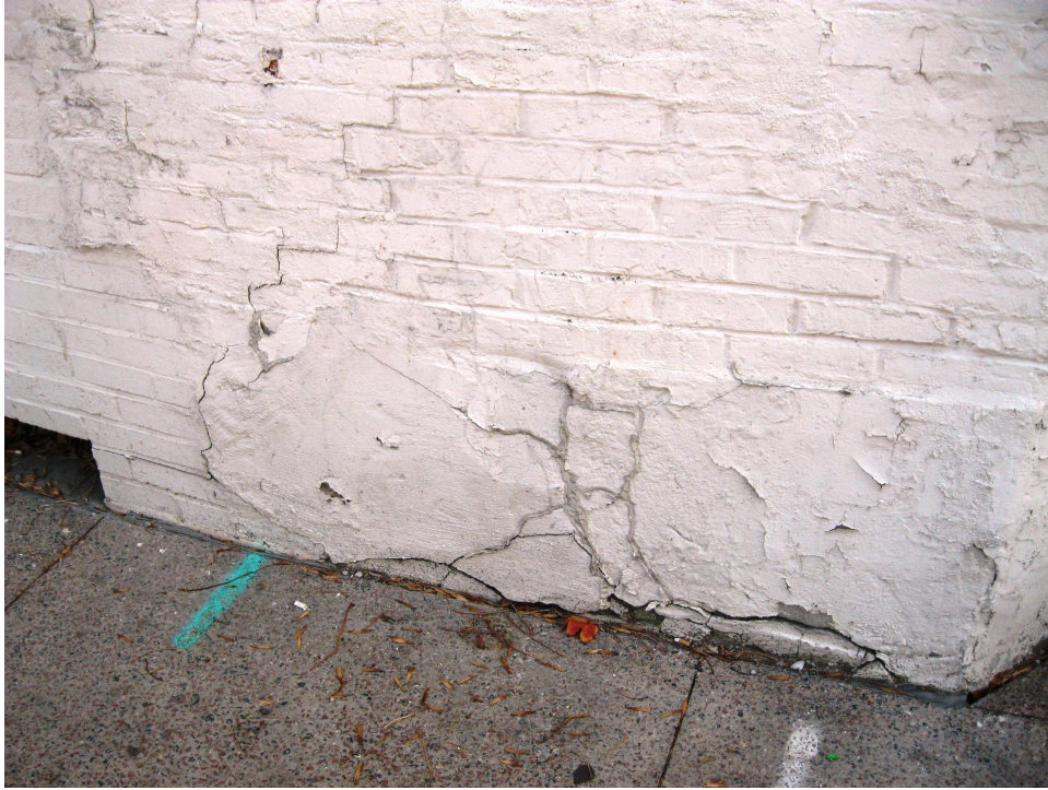
Photo 11 – Exterior wall base at Fairchild Street sidewalk
