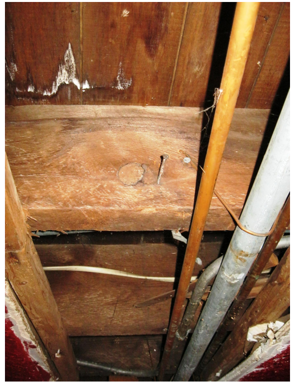
Photo 6 – 1 st floor joist framing
