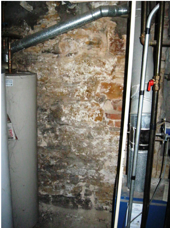
Photo 9 – Basement wall along Fairchild Street
