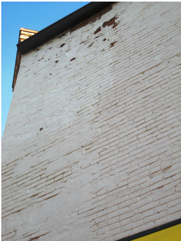
Photo 3 – Fairchild Street elevation at corner
