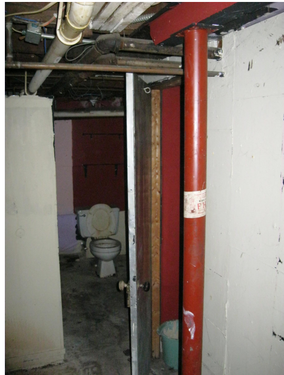
Photo 10 – 1 st floor shoring beam and post
