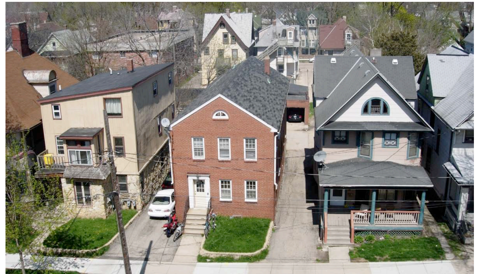
View of 119, 123 & 125 from the Capitol North Ramp
