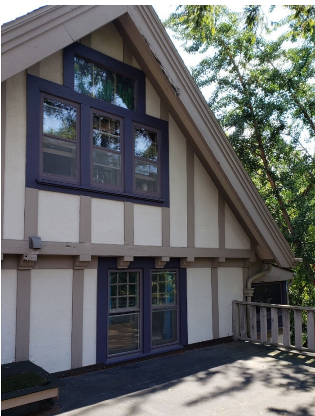
Second Floor West Addition Lkg SE
