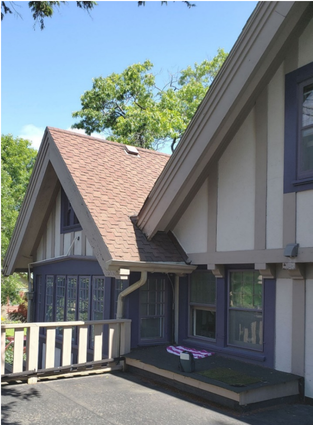
Second Floor West Addition Lkg NE
