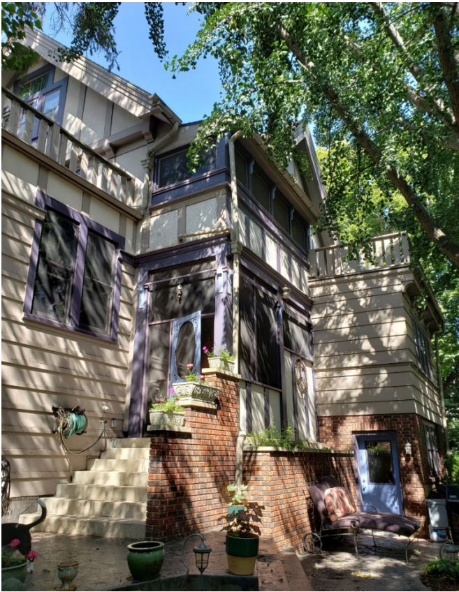
West addition and South Side Lkg North East
