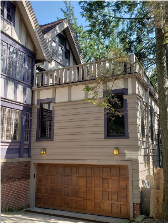
West Living Room/ Garage Addition Lkg South
