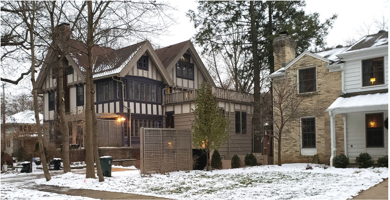
View from W. Chadbourne Lkg SE
