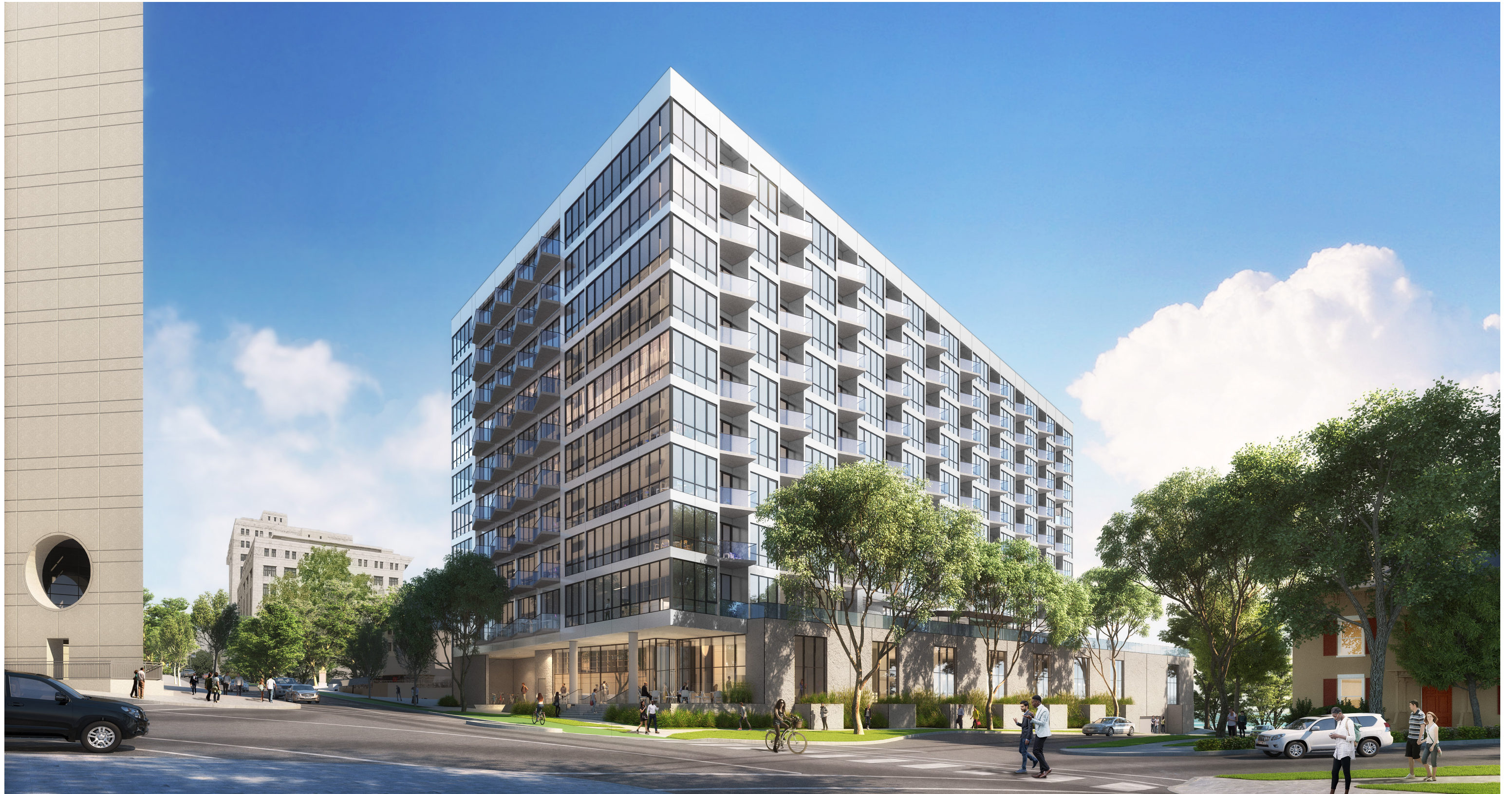
WILSON ST. + HENRY ST. LOOKING EAST
