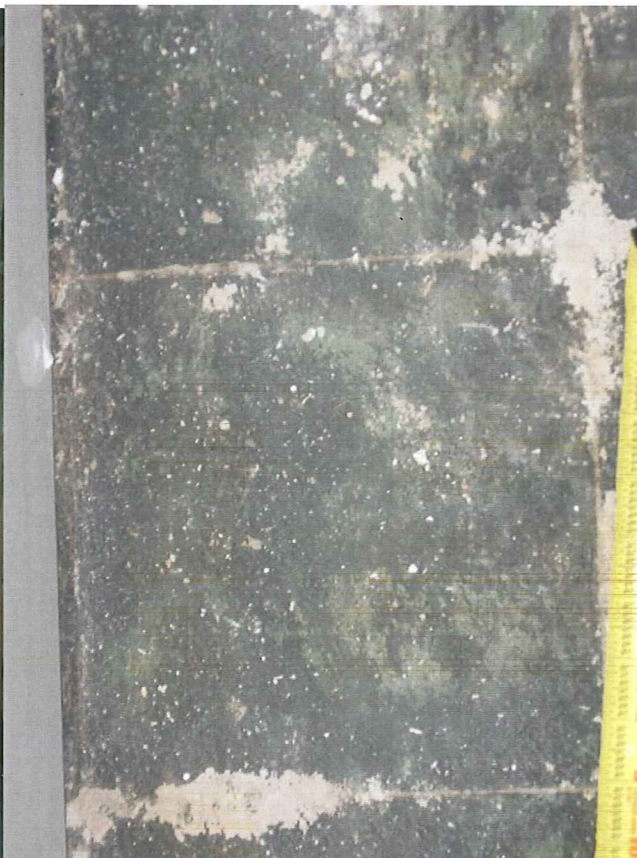
4908 Asbestos tile floor
