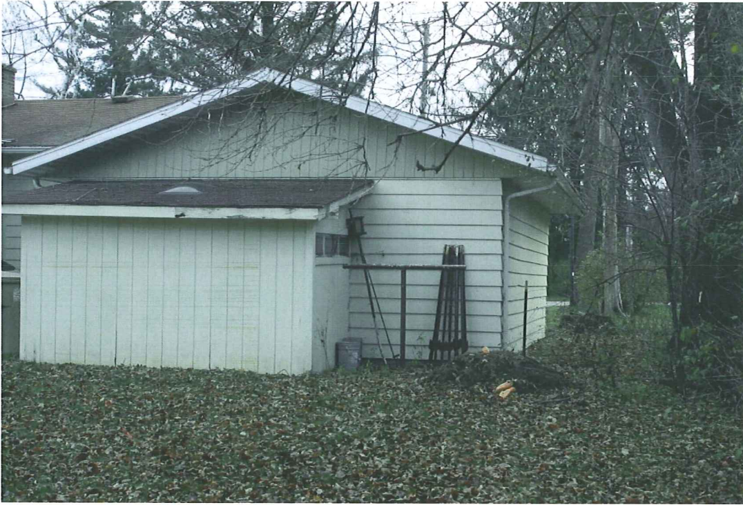
4908 Back of garage
