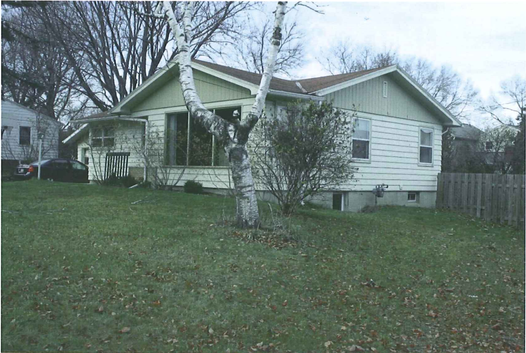
4908 Southeast corner facing Pacific Cycle
