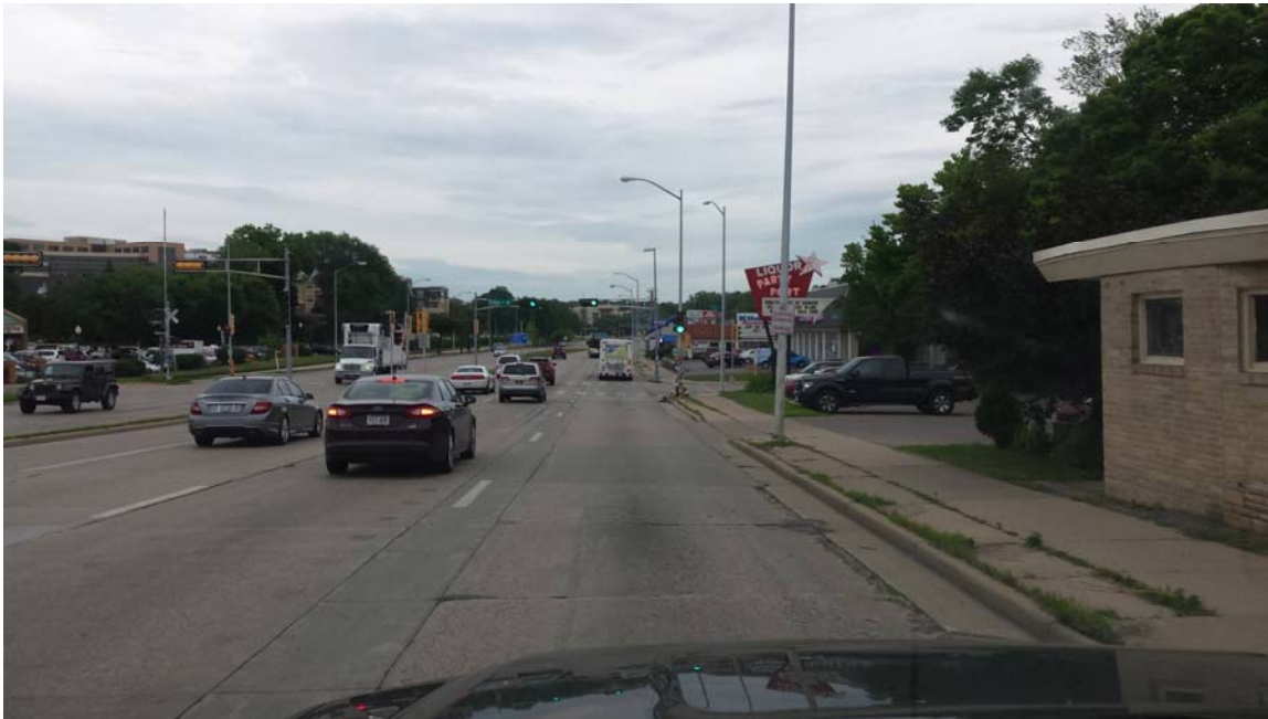
Looking East towards Ridge St. approx. 170 West of Stop Bar Signal indications are Green
