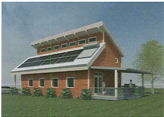
Southeast View - Rear of House
