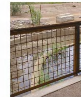
GUARDRAIL FENCE WELDED WIRE FENCE AT RETAINING WALLS
