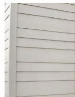
CEMENT BOARD LAP SIDING HARDI-PLANK LAP SIDING OR SIM. SMOOTH FINISH ALTERNATING 4" AND 8" PLANKS
