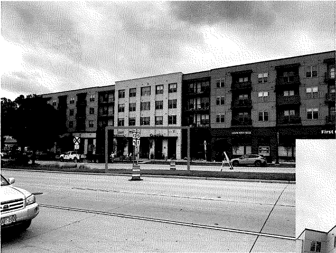
View from Park looking East
