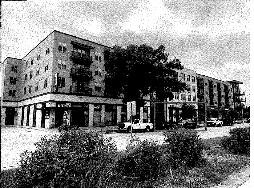
View from street looking South
