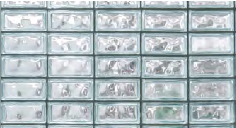
GLASS BLOCK - CLERESTORY WINDOWS AT BASE
