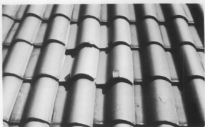
Repairs on this pantile roof were made with new tiles held in place with metal hangers. (Main Building, Ellis Island, New York)
