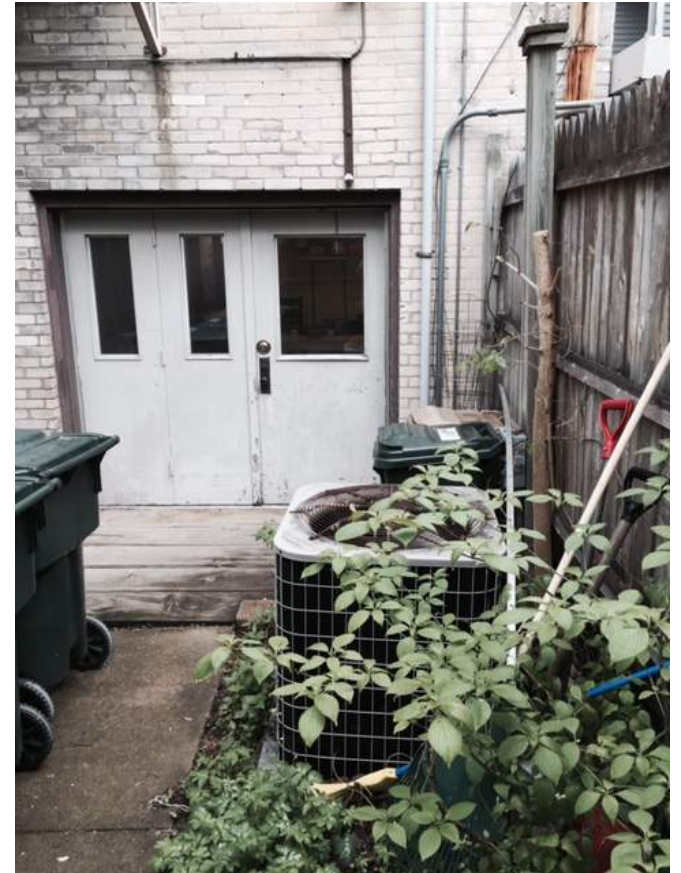
Rear of 409 E. Main Street
