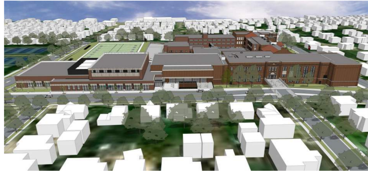
C AERIAL VIEW OF ATHLETIC ADDITION - BASE
