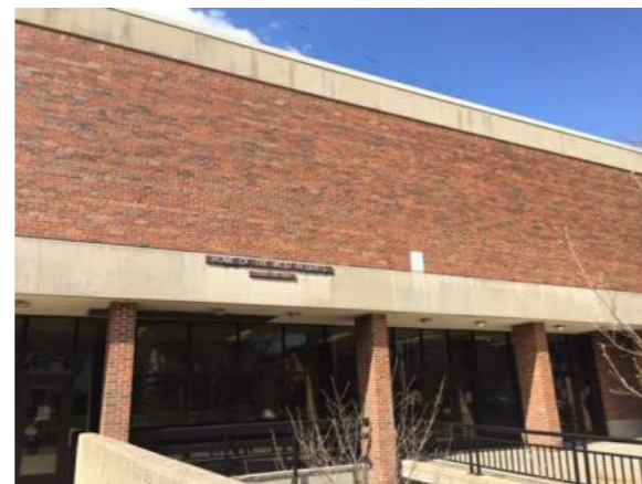
EXISTING BRICK AT GYM
