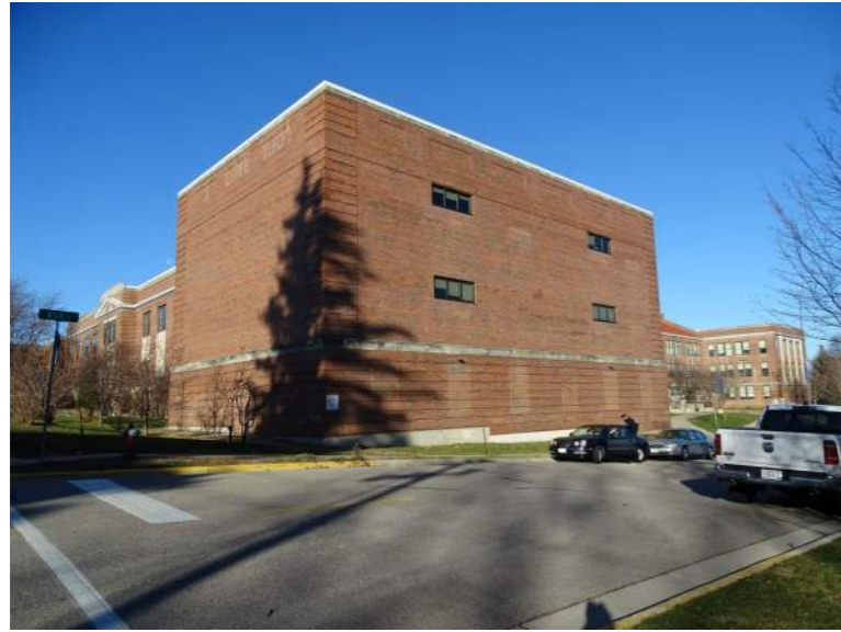
1. VIEW AT THE CORNER ASH STREET AND REGENT STREET
