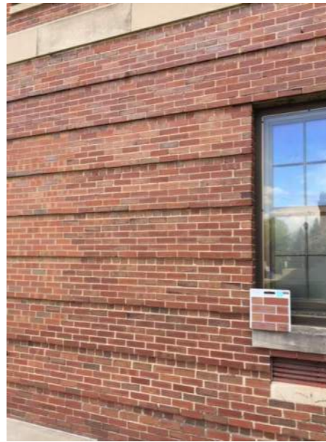
EXISTING BRICK AT WELCOME CENTER
