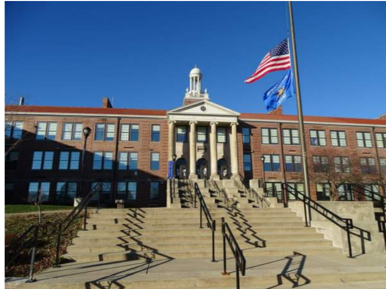
2. VIEW OF ASH STREET ENTRANCE
