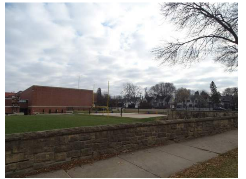
6. VIEW TO WEST GYM
