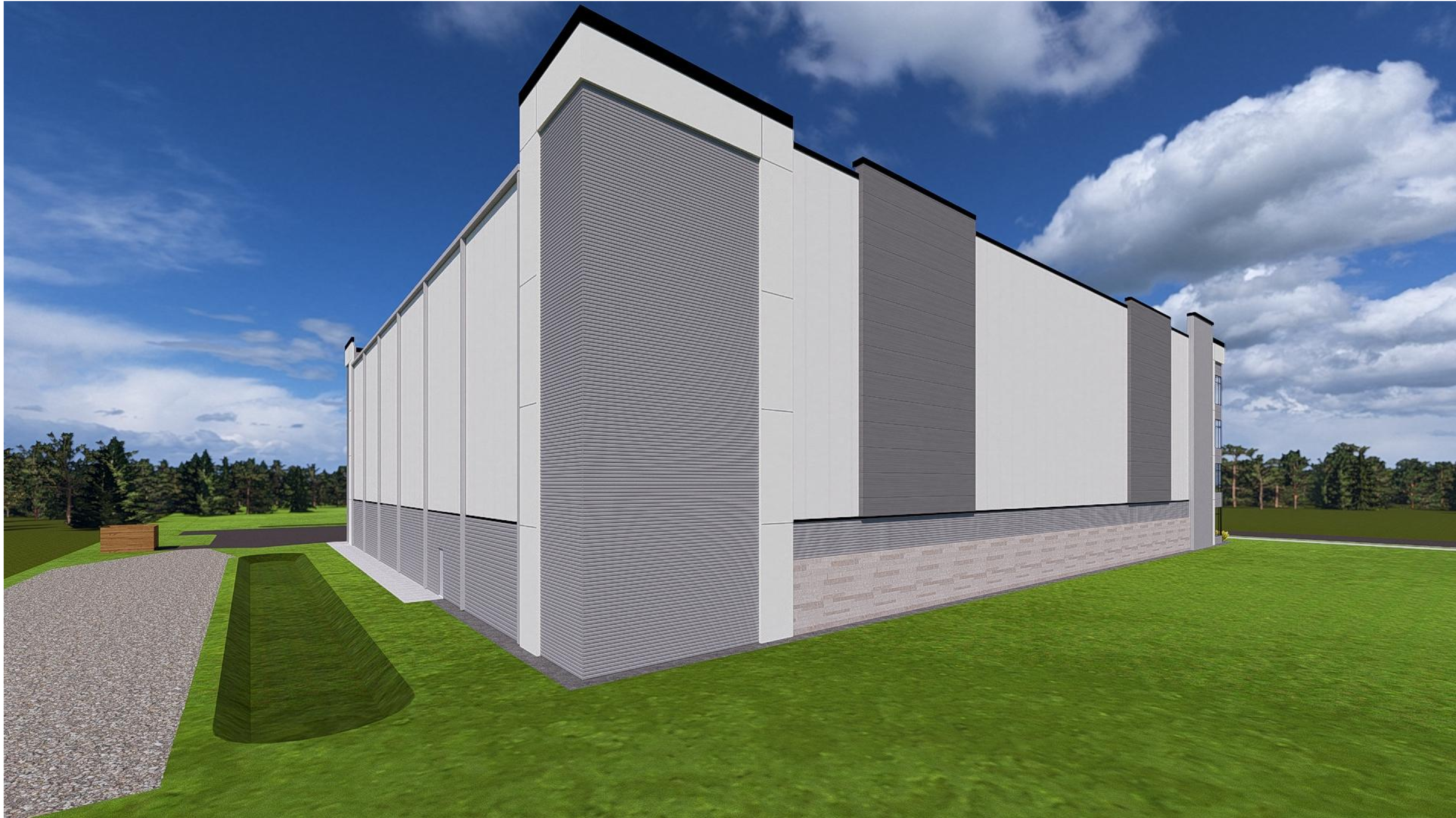
Southwest Corner | Back
