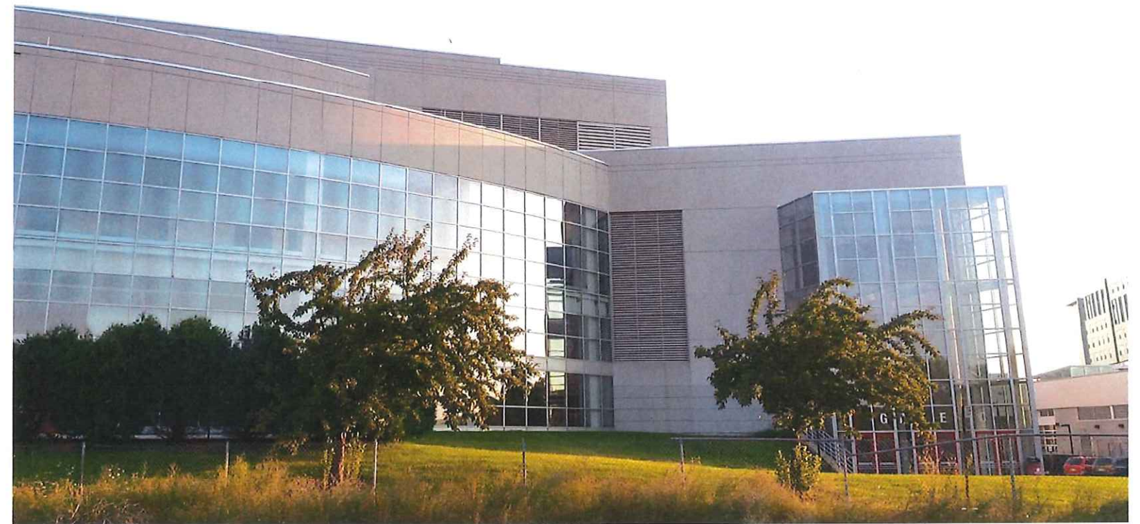
Existing southeast corner/facade view from commuter bike path
