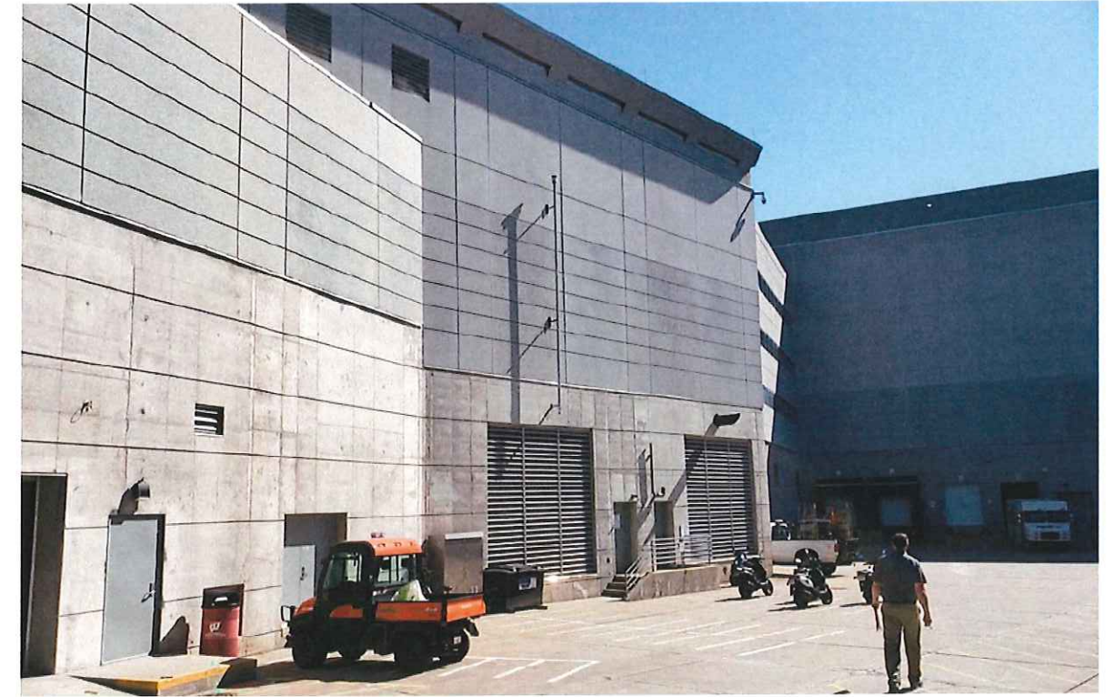
View into Kohl Center loading area
