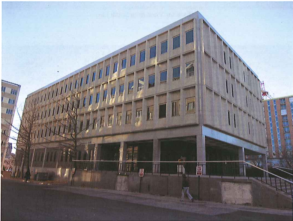
Exterior View from Northwest
