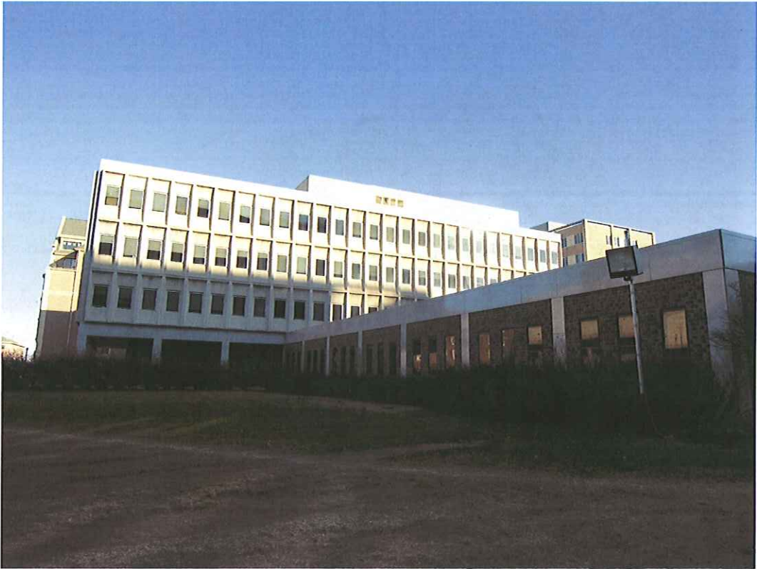
Exterior View from Southwest (close-up)
