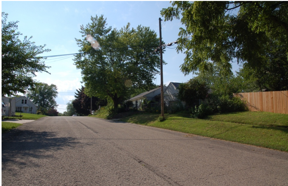
Town of Blooming Grove street with no curb and gutter
