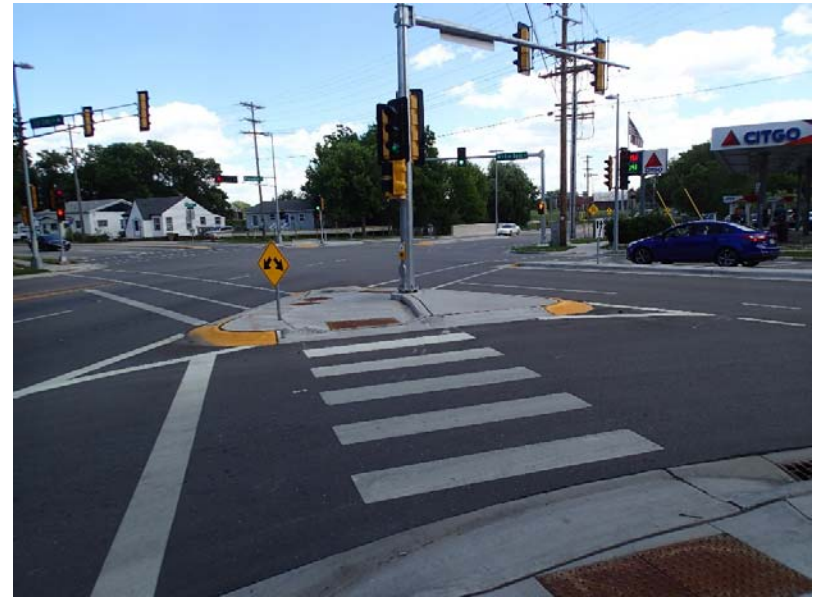
Continental crosswalk at Fair Oaks/Milwaukee Street intersection
