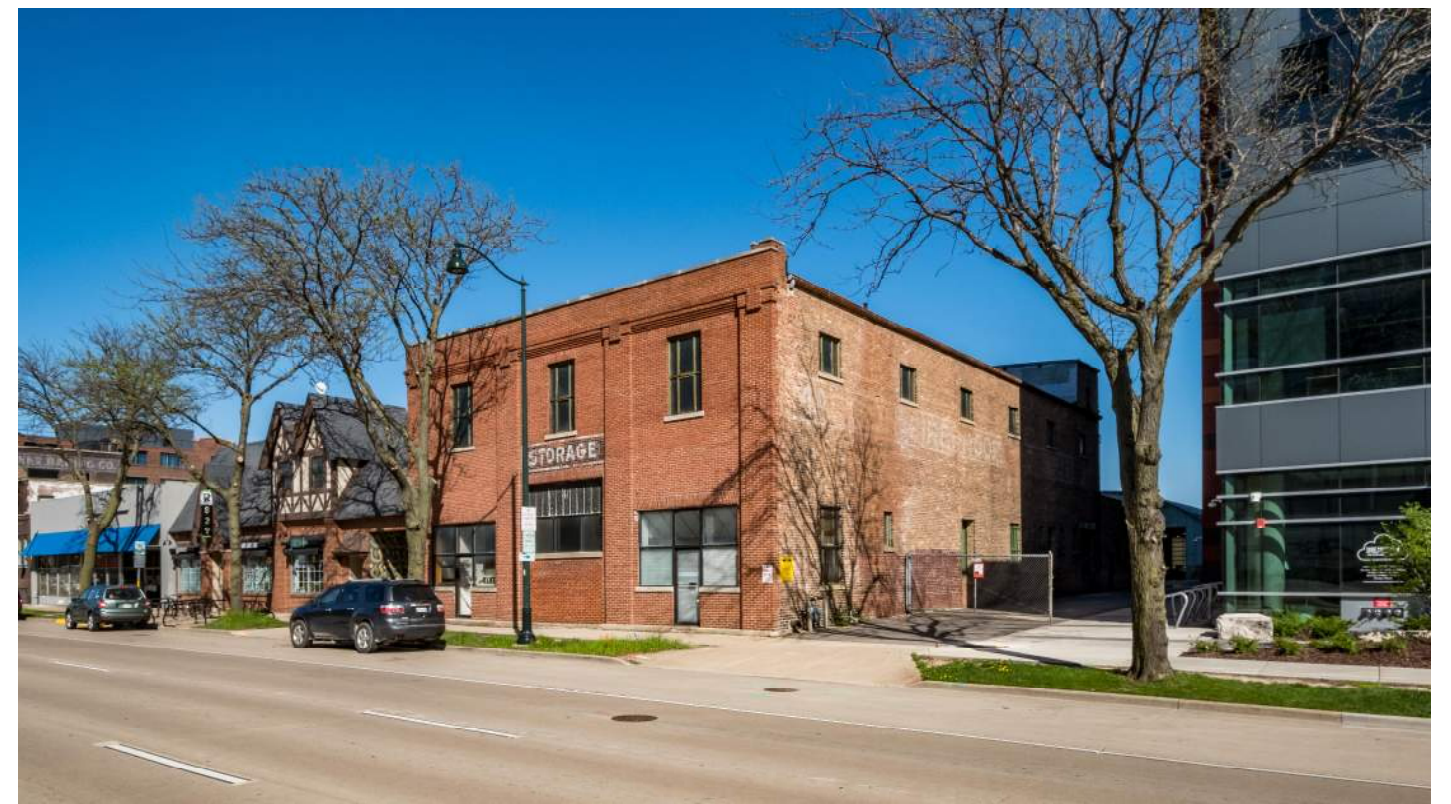
Image No. 2 Looking East
