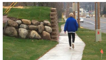
New sidewalk along Buckeye Road.
