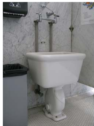
Figure 27 – Slop Sink in Women's Restroom
