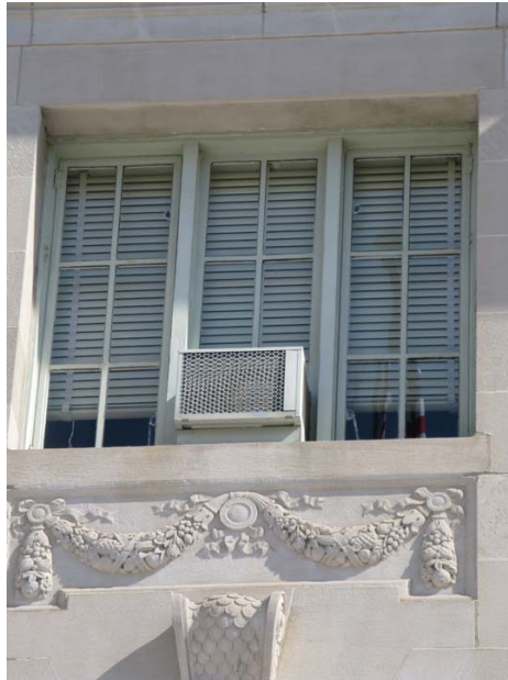
Figure 63 – Steel Window with Stone Carving Decorations
