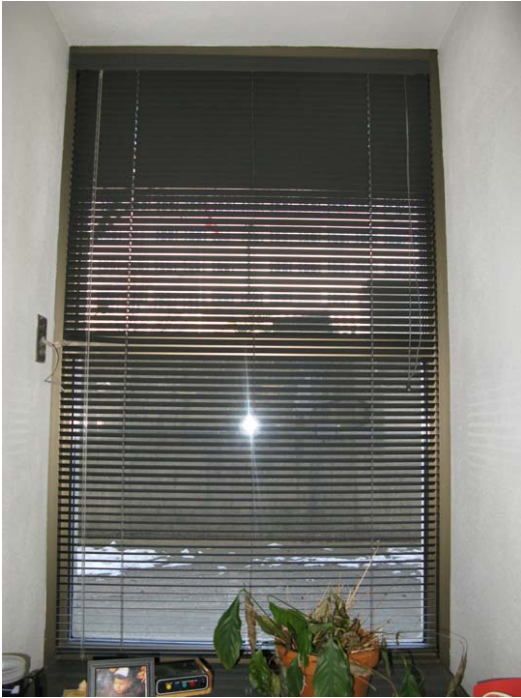
Figure 15 – Aluminum Framed Replacement Windows are Located on the Lower and First Floor Levels
