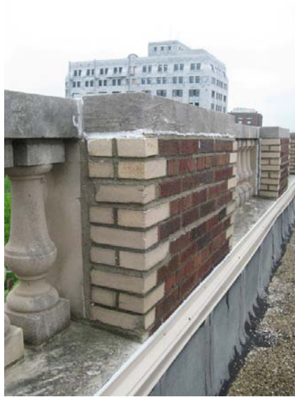
Figure 62 – Brick and Stone Parapet
