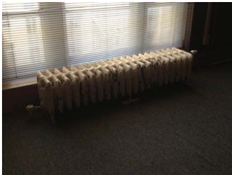
Figure 35 – Steam Radiator
