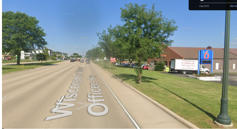
Figure 4. – E. Washington Ave Wide curb pan/bike lane
