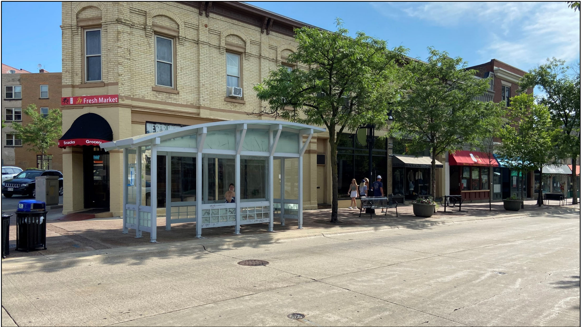
State Street at Gorham Street, View Northeast – Existing Within State Street Historic District
