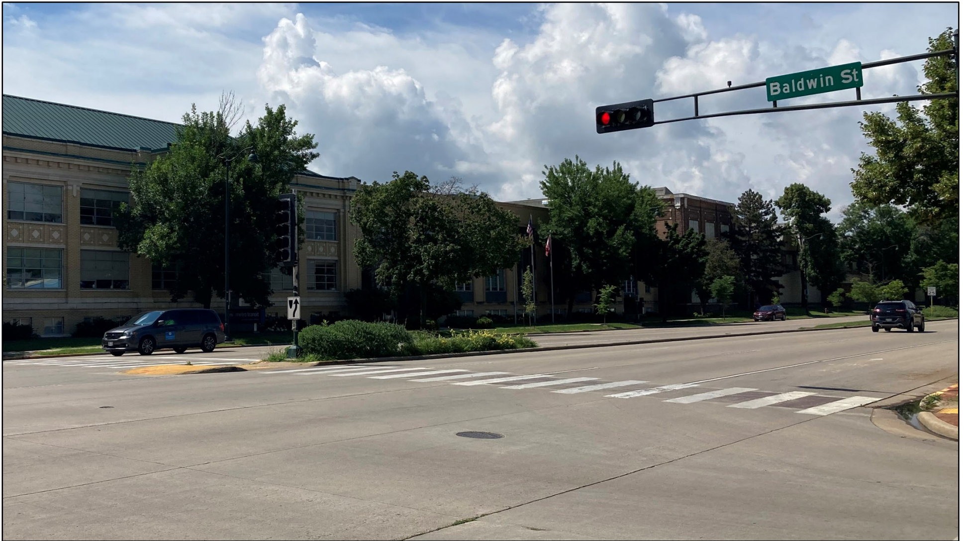
E. Washington Avenue at Baldwin Street, View South – Existing Adjacent to Gisholt Machine Company
