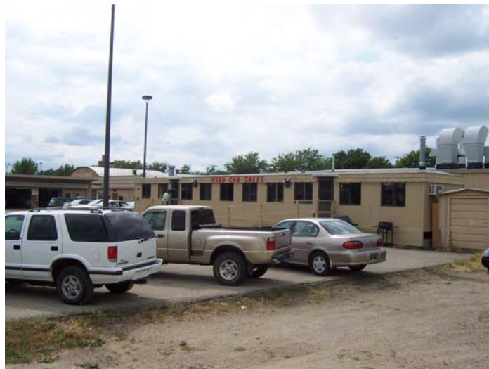
West – Used Car Sales Office
