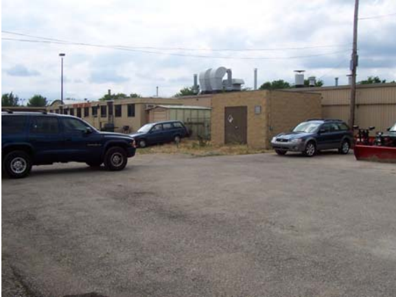
West – Used Car Sales Office
