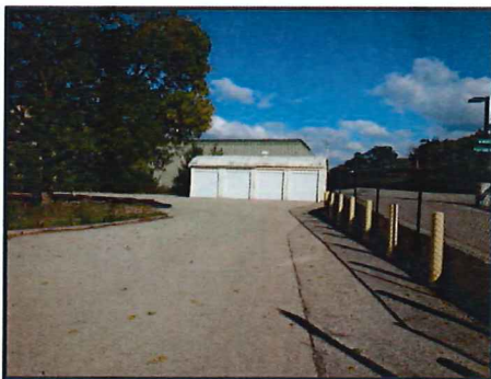
Exterior- Driveway Approach to Rear, Also Showing 4 Bay Garage
