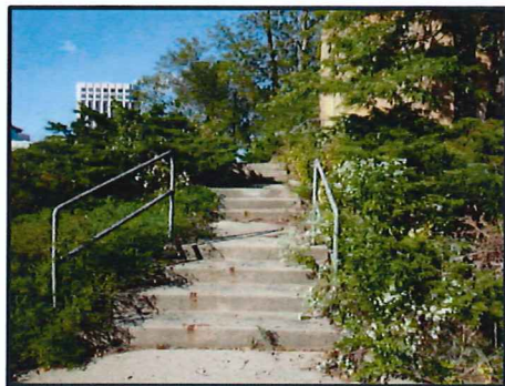
Exterior- Front Stairwell
