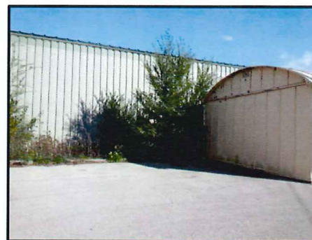
Exterior- Side of Detached Garage
