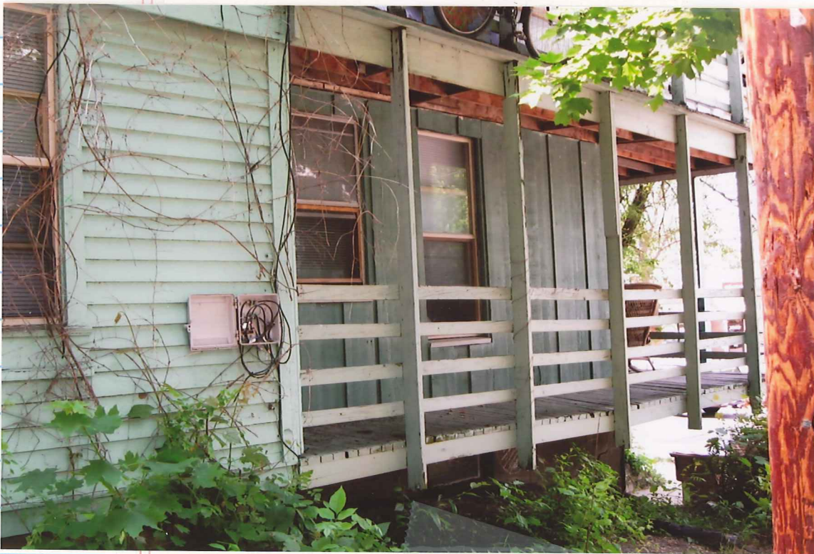
1st floor deck from Brearly St
