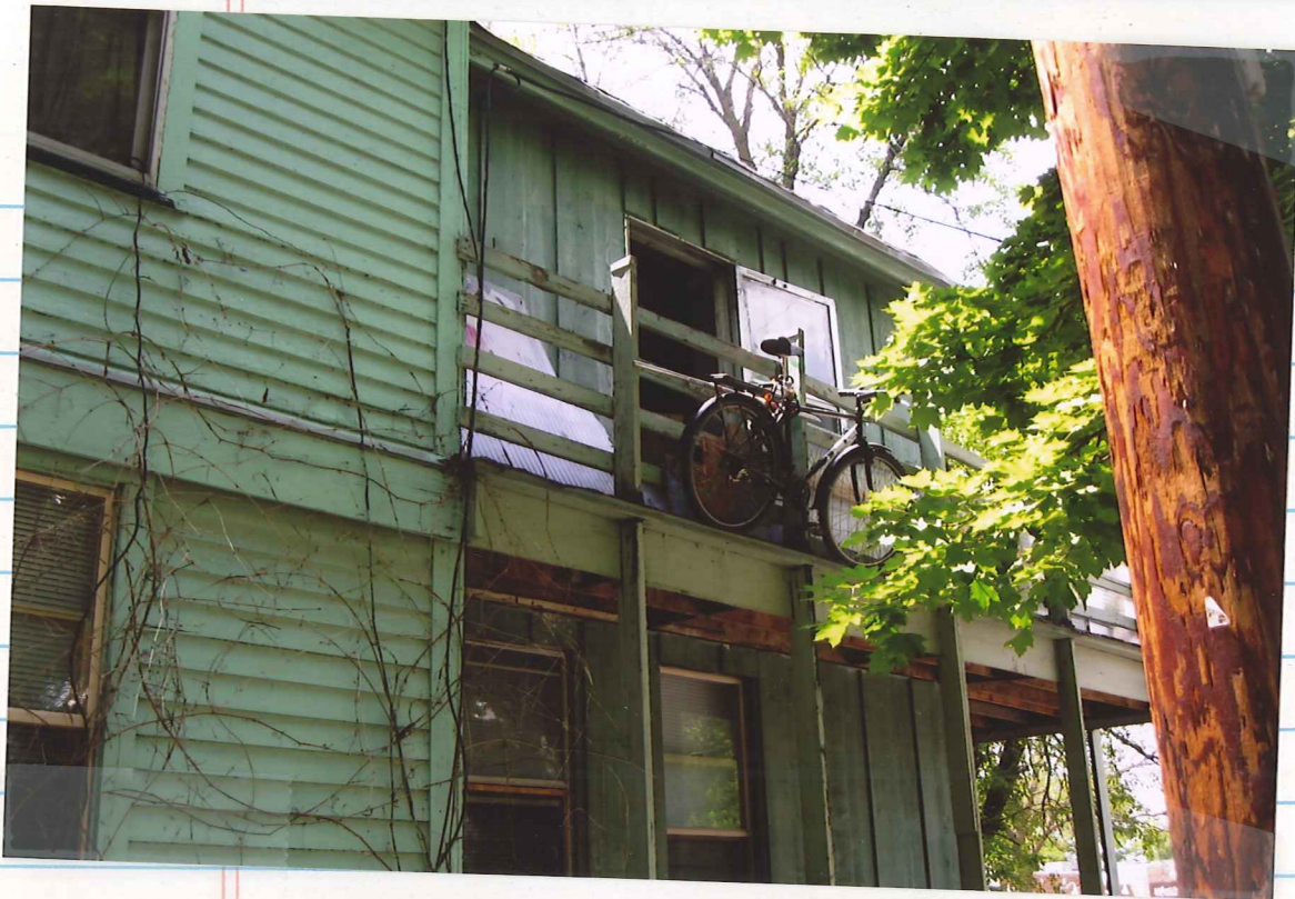
2nd floor deck from Brearly St (note door)
