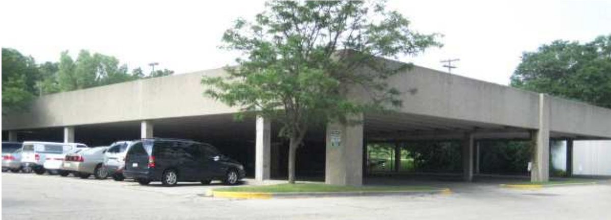
610 N. Whitney Way, "PSC Parking Ramp"
