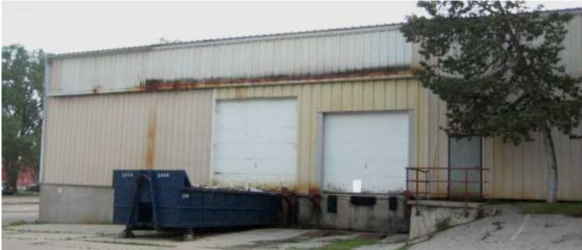
5107 University Avenue, "Lower Warehouse".
