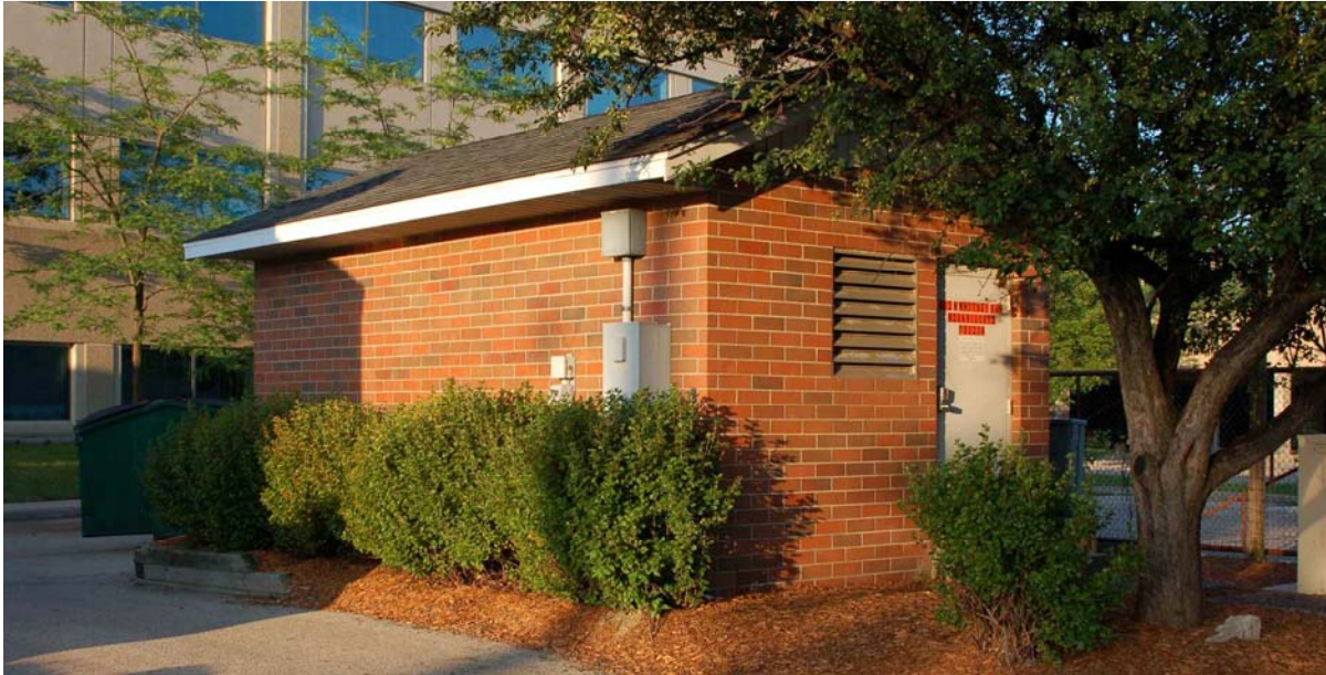
Easement, "AT+T Utility Shed"
