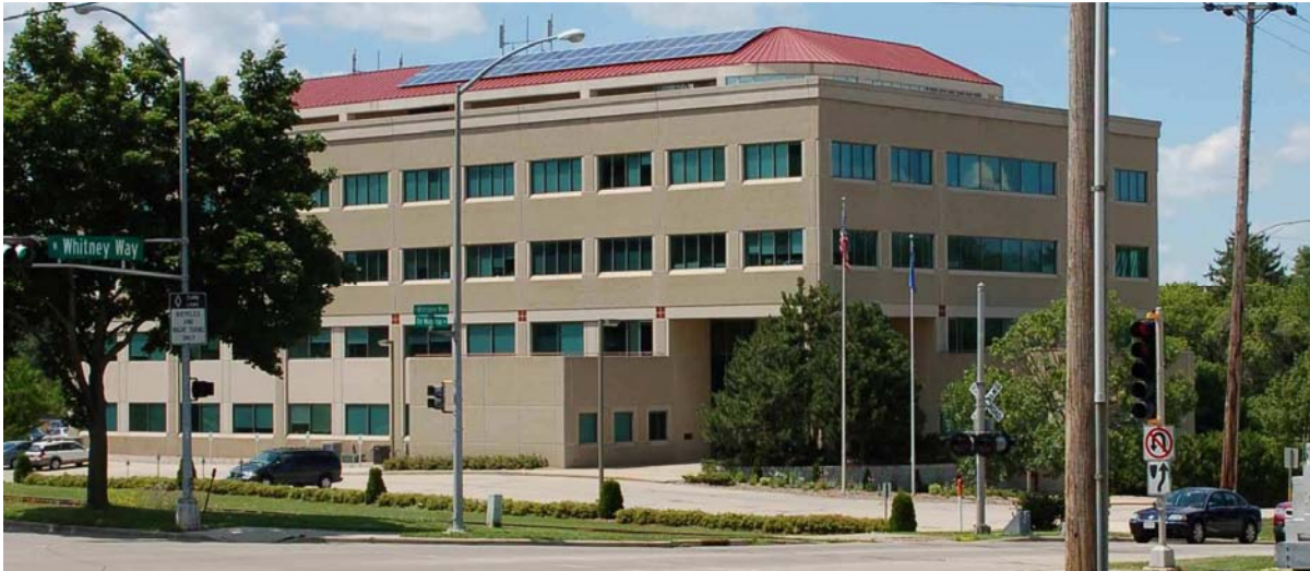
610 N. Whitney Way, "PSC Building"
