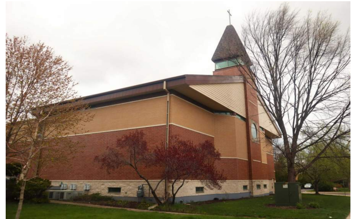
2004 construction, South and East facades
