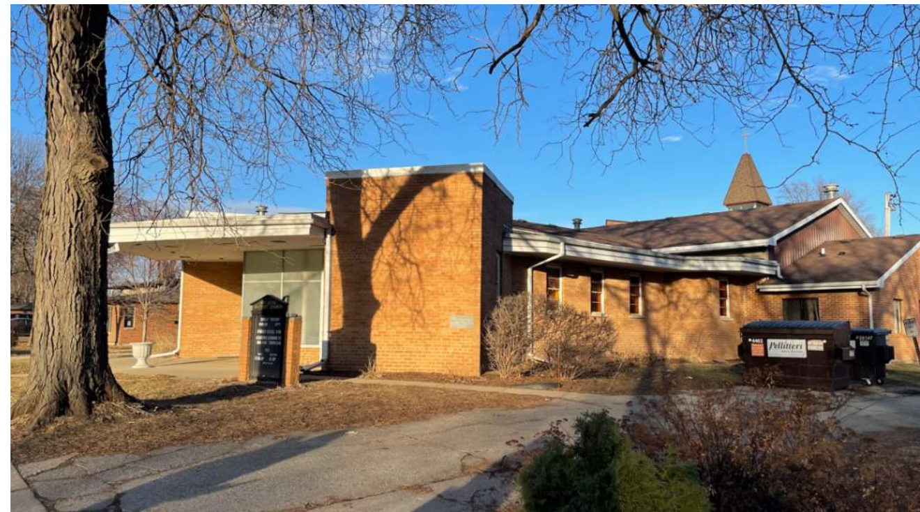
1961 construction, Southwest facade
