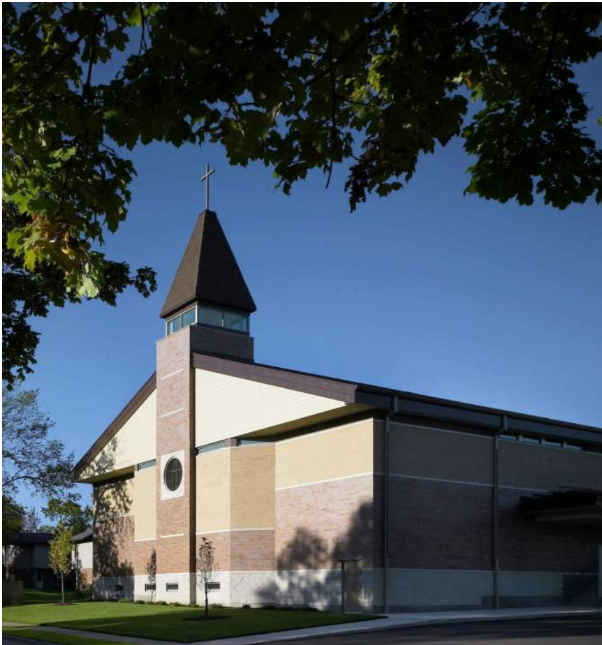
2004 construction, East and North facades
